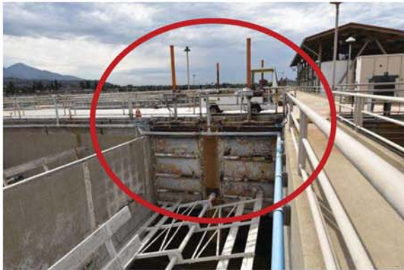
Photo 3. Inlet Gates and Associated Actuators at Basin No.1 (Sedimentation Basin), Facing West.
