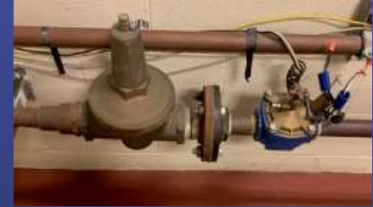
Master Valve Replacement
