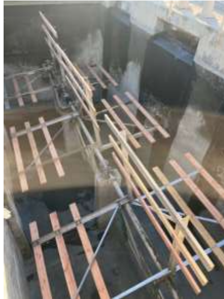
Installation of new flocculator paddles at the Diemer Wash Water Reclamation Plant
