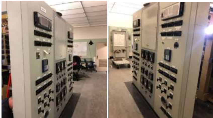
Installation of new protection panels for an upgraded transformer bank at Eagle Mountain pumping plant
