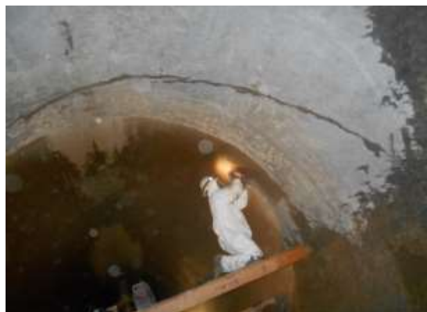
Staff prepping Lakeview Siphon repair area for installation of internal rubber seals and metal bands
