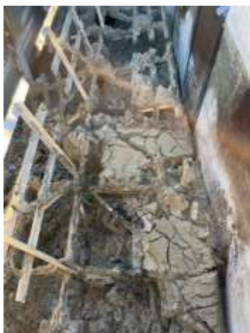
Sludge and coal accumulation in a flocculation basin at the Diemer wastewater reclamation plant
