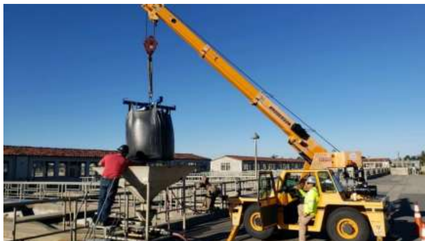
Staff unload a one-ton bag of filter media into a hopper at the Weymouth plant
