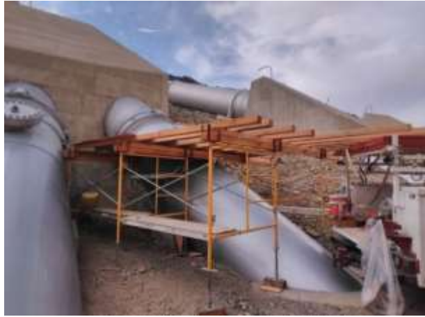
Scaffold construction for recirculation pipe assembly installation at Eagle Mountain pumping plant
