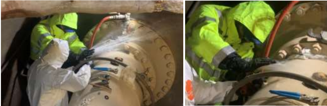
Staff successfully replacing a venturi access port fitting at the FM-01 service connection
