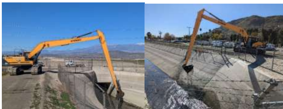
Staff using a long reach excavator to clean the San Diego Canal
