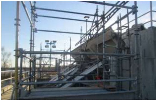
Welded reinforcing beams on San Diego Canal radial gate to reduce vibration
