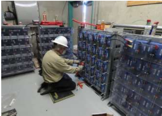
Staff installing new pumping plant station battery banks
