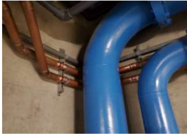
Copper piping joints after replacement with crimps at the Skinner plant
