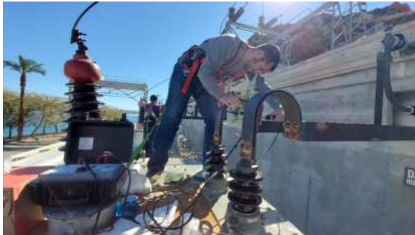
Class of 2023 electrical apprentice performing contact resistance testing at Whitsett pumping plant
