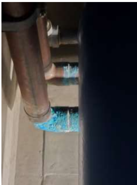
Corroded pipe in hard to reach corner at the Skinner Plant
