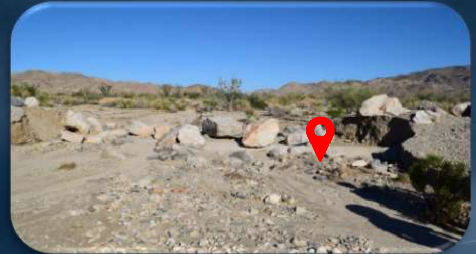
Exposed conduit at Pinkham Wash October 2018
