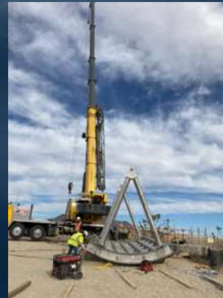
Installation of new radial gate on CRA in 2020
