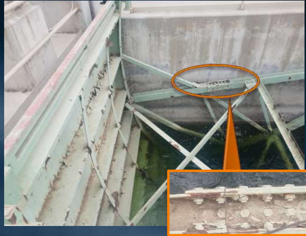
V-08 radial gate partially submerged in water
