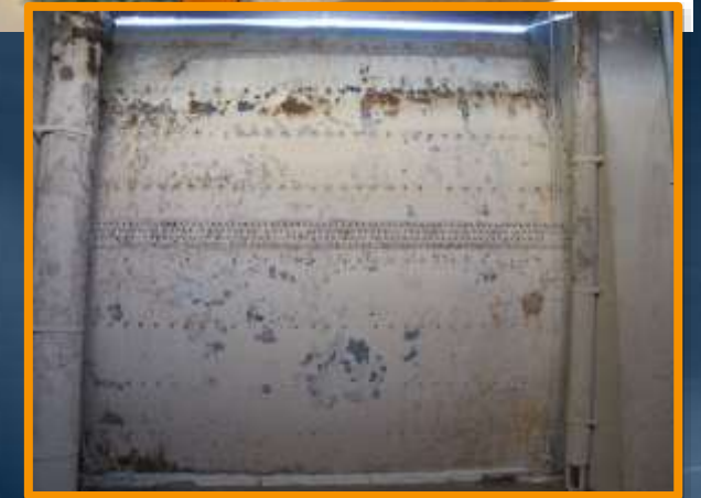
Corroded Radial Gate
