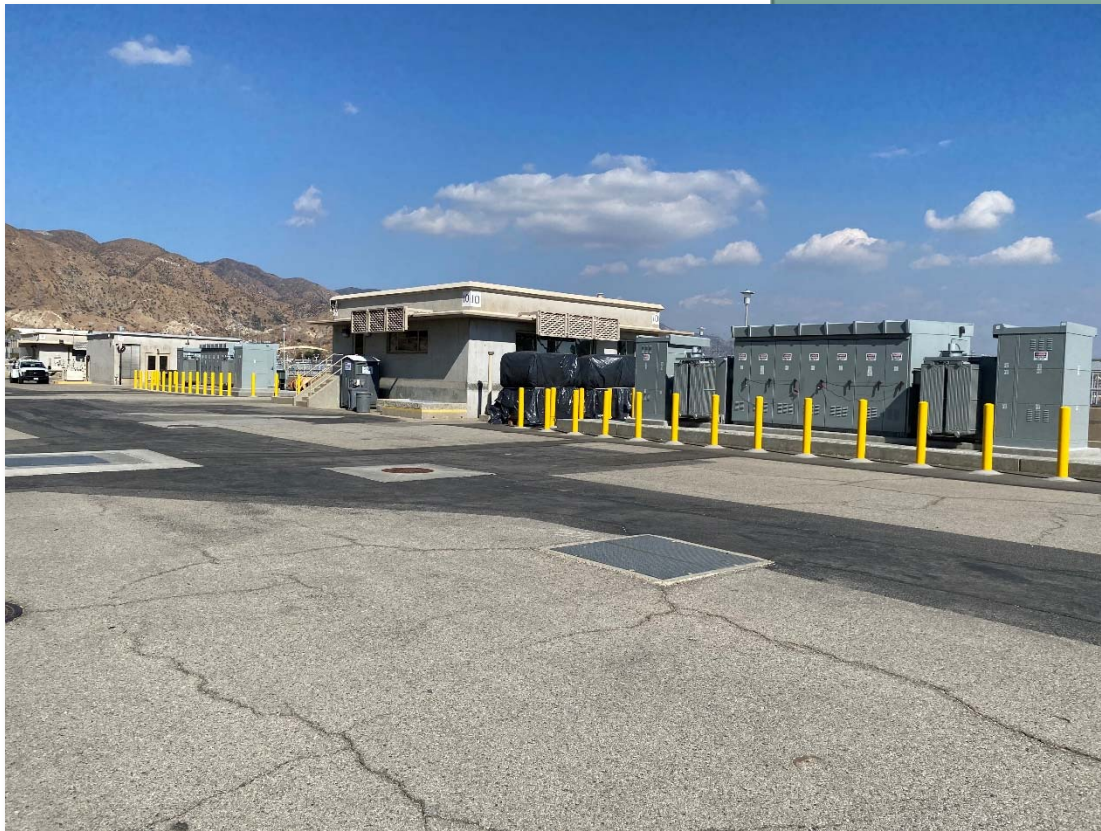
Completed unit substations at the Jensen plant
