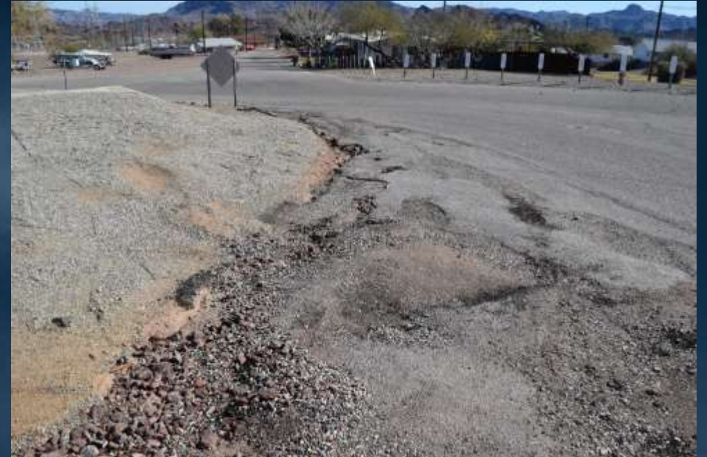
Deteriorated asphalt pavement at Gene Pumping Plant
