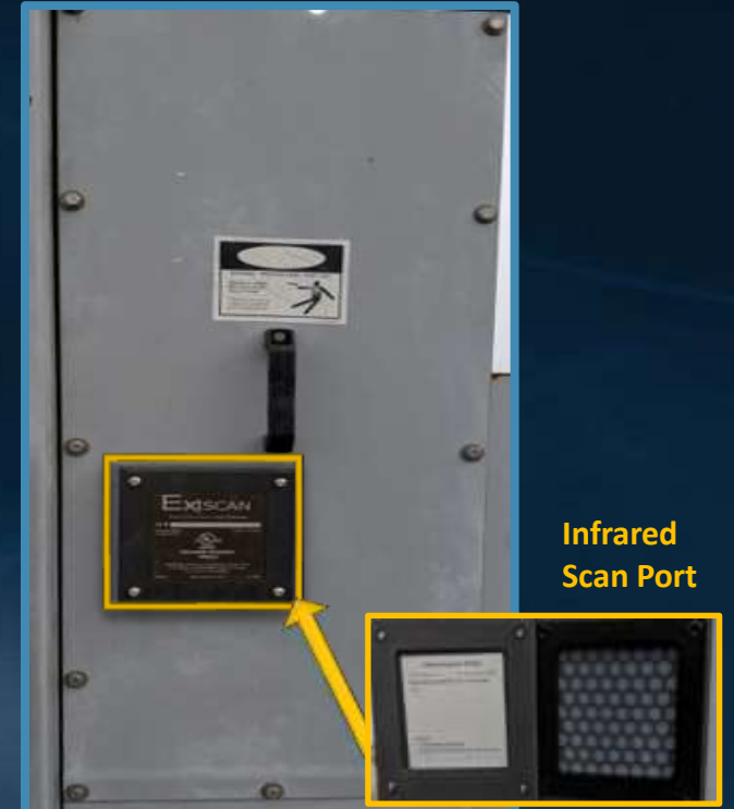
Diemer High Voltage Scan Port Installation
