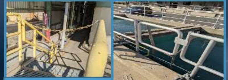
Diemer Chains replaced with Swing Gate
