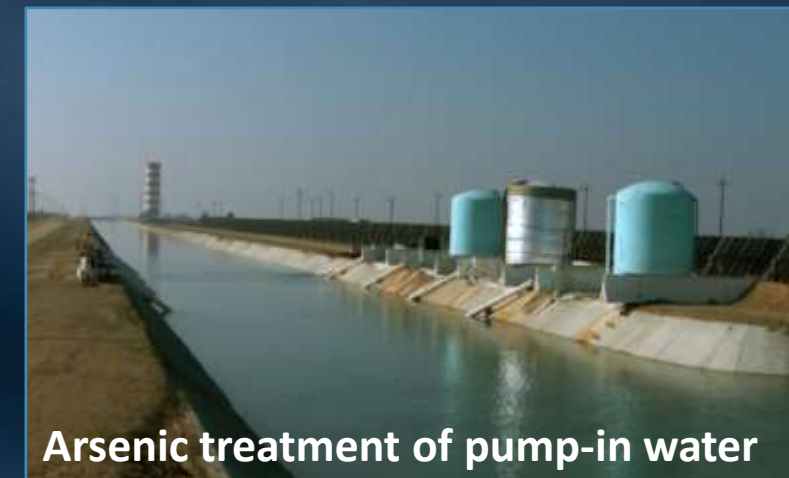
Pump-in along CA Aqueduct
