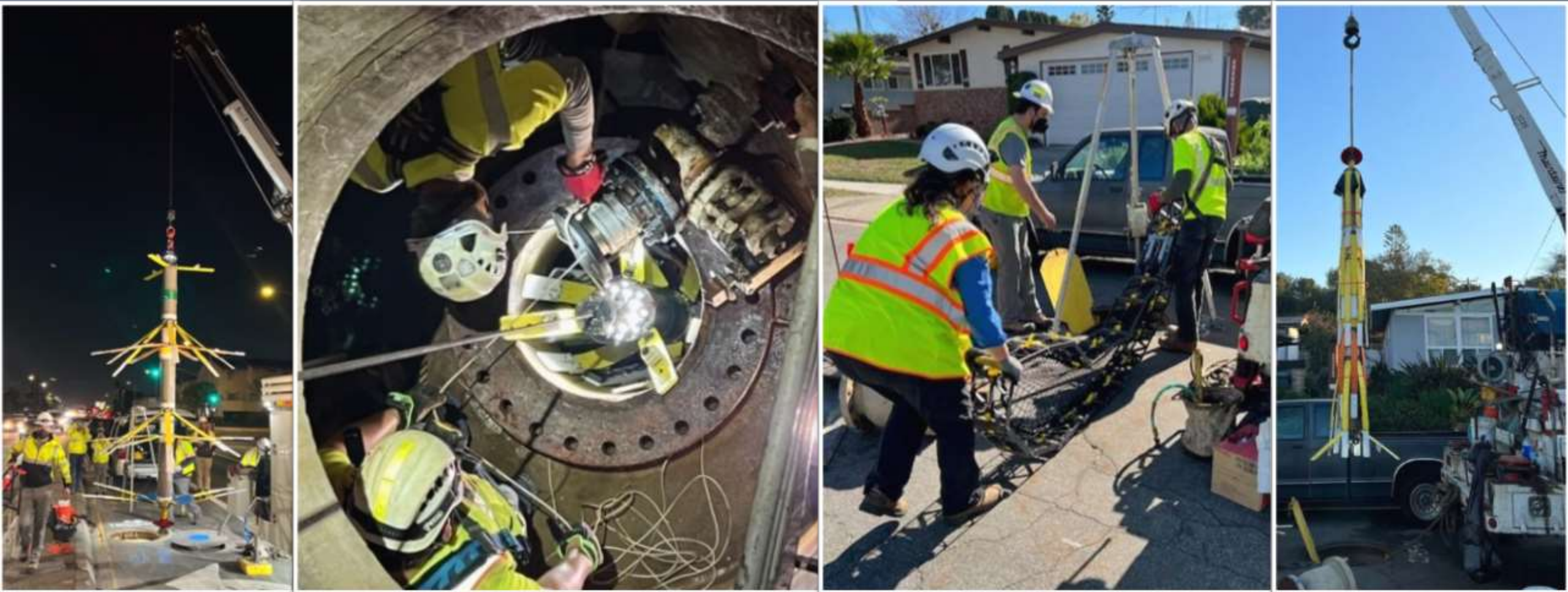
Placing the PipeDiver, setting up the catch net, and removing the PipeDiver
