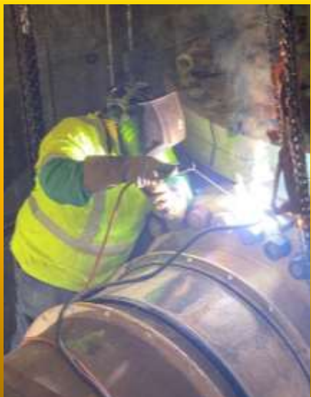
Staff Welding Lifting Eyes
