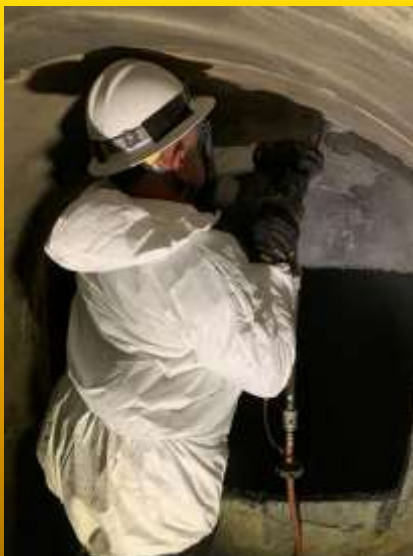
Staff Removing Bulkhead
