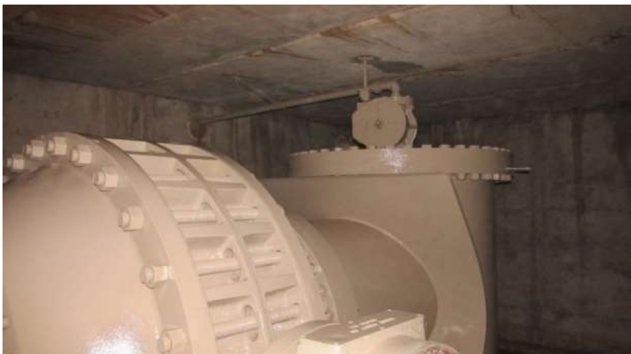
Service connections OC-68 and OC-69 structure after coating maintenance
