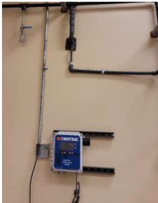
Particle counter mounted on the wall near the SCADA system signal tie-in at the Weymouth plant
