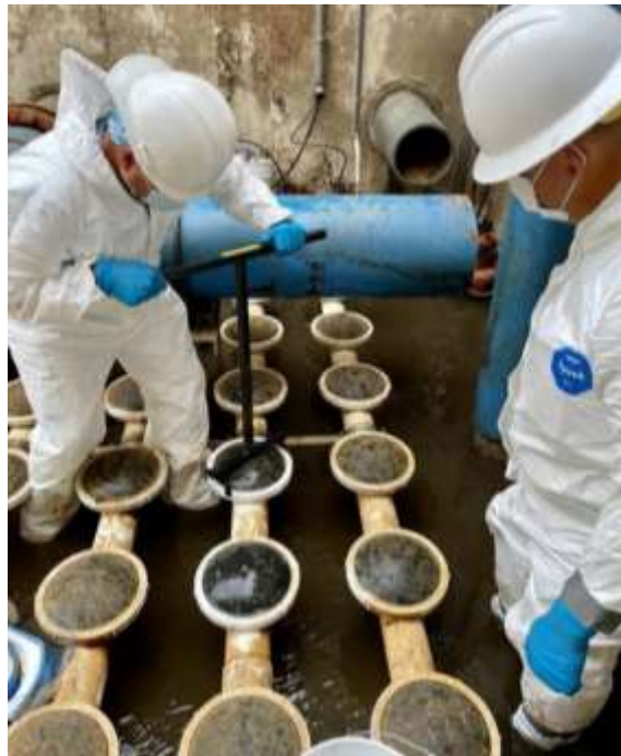
Staff replacing a damaged diffuser membrane in the aerobic biological tank at the demonstration facility
