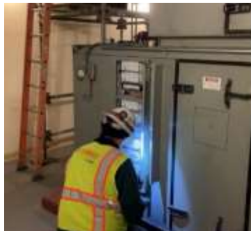
Headquarters Building Improvements—Installation of UVC light controls in HVAC system
