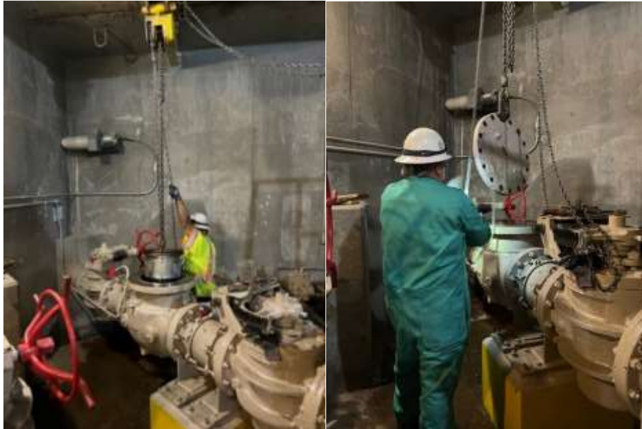
Staff installing internal globe valve components (left) and cover flange (right) at the Cohasset PRS on the East Valley Feeder
