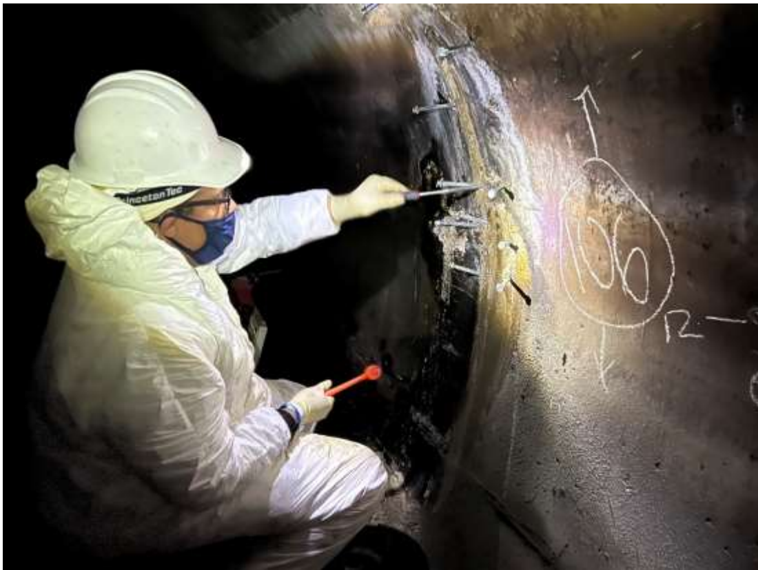
Staff preparing for hydrophilic injection repairs of the Rainbow Tunnel
