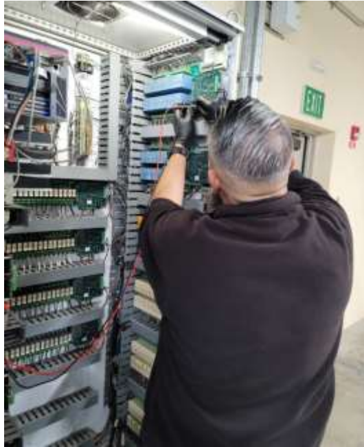
Staff testing loop integrity at the RTU for the particle counter at the Weymouth plant
