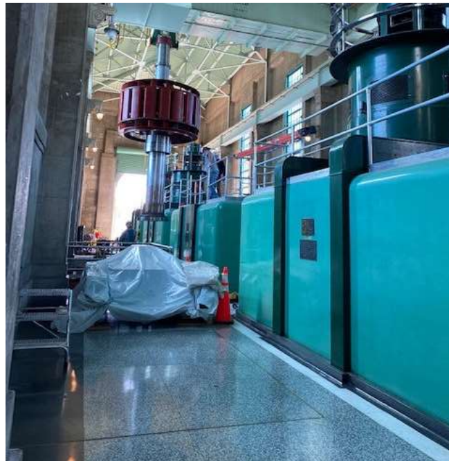
Staff installing the rotor on a pump unit at Gene pumping plant
