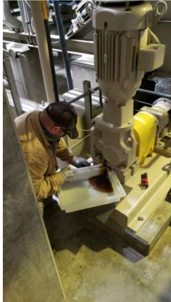
Staff performing lockout/blockout of a pump for maintenance (left) and staff performing a pump oil change at the Weymouth plant
