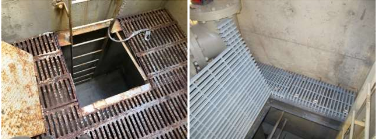
Corroded grating (left) and new fiber-reinforced polymer grating (right) at the Lower Feeder blow-off structure
