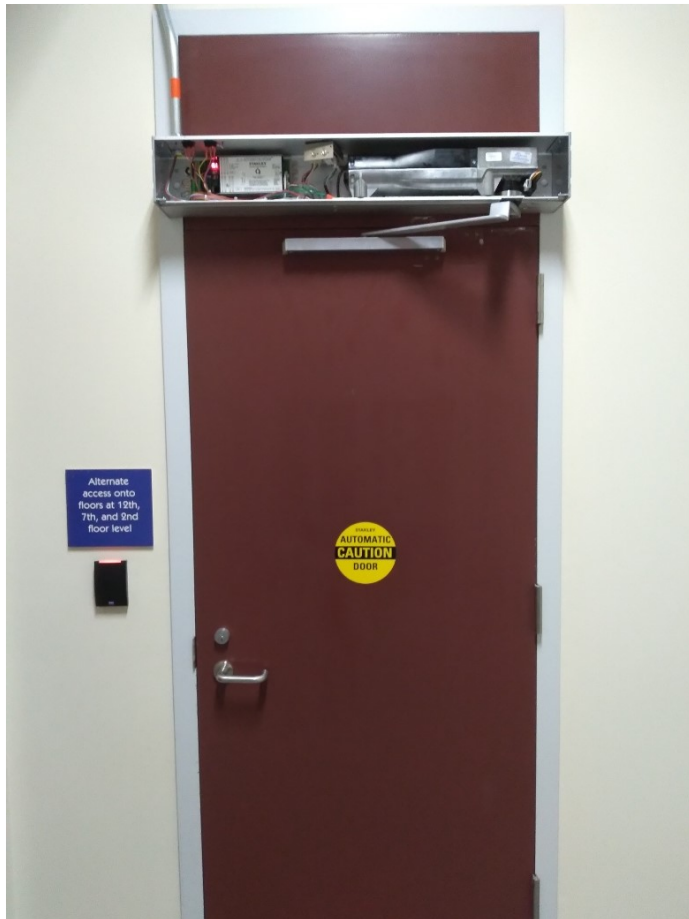
Installation of power door assist mechanisms
