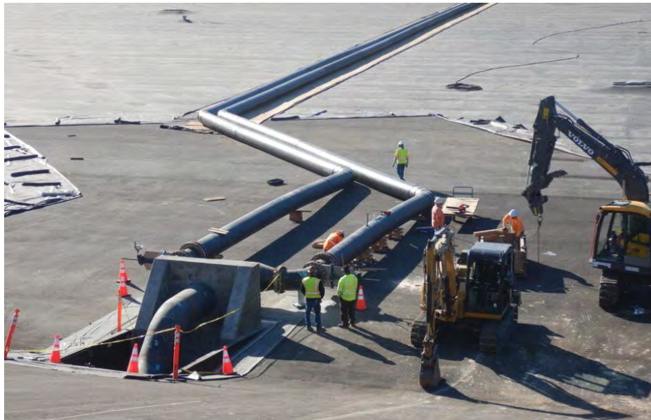
Second Lower Feeder PCCP Rehabilitation Reach 3B —Installation of a temporary bypass line at Palos Verdes Reservoir needed for an upcoming Second Lower Feeder Reach 3B shutdown
