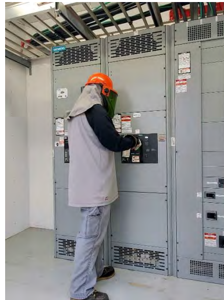
Staff verified amperage (left) and performed a lockout/blockout (right) at the Napolitano Innovation Center
