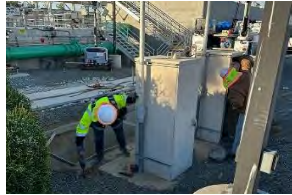
Existing meter (left) and staff preparing to replace flow meter (right) at EM-04 service connection
