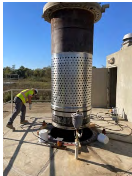
Staff lifting a sleeve valve at the Auld Valley Pressure Control Structure
