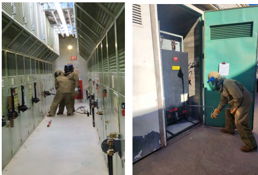
Staff performed high-voltage switching (left) and isolate and lock (right) a 6.9kV circuit breaker
