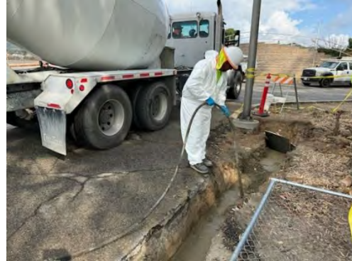
Staff placing electrical encasement
