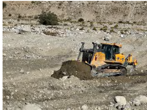
Staff utilizing an excavator (left) and a dozer (right) to repair the berm
