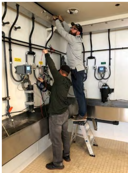
Staff installed water temperature probe at the ozone building laboratory at the Skinner plant
