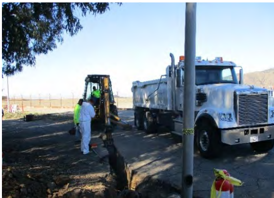
Staff excavating for new conduit (left) and performing circuit repairs (right)
