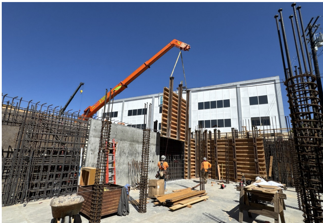
Sepulveda Feeder Pump Stations – Installation of Basement Wall Forms in Electrical Building
