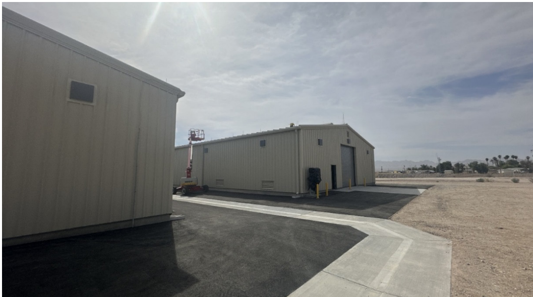
CRA Storage Buildings – Contractor Installing Lightning Protection System at Iron Mountain
