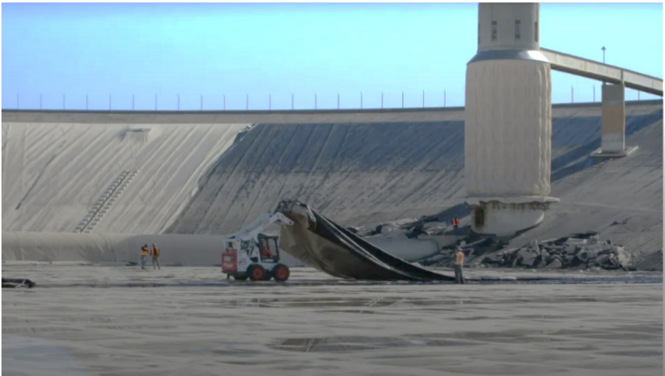
Garvey Reservoir Rehabilitation — Demolishing Existing Cover and Rain Collection System
