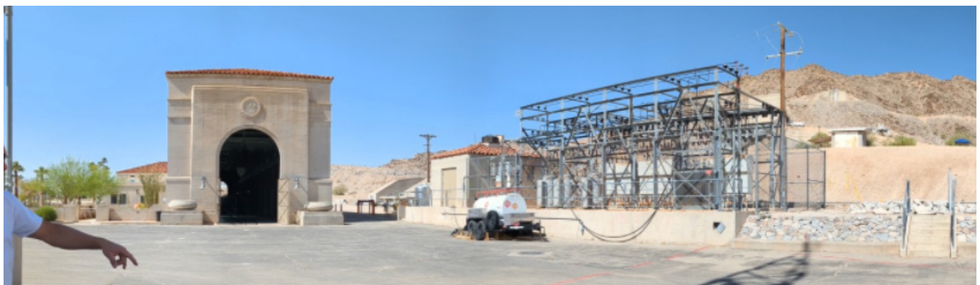
Iron Mountain Pumping Plant – Pump House & 2.4 kV Switchrack
