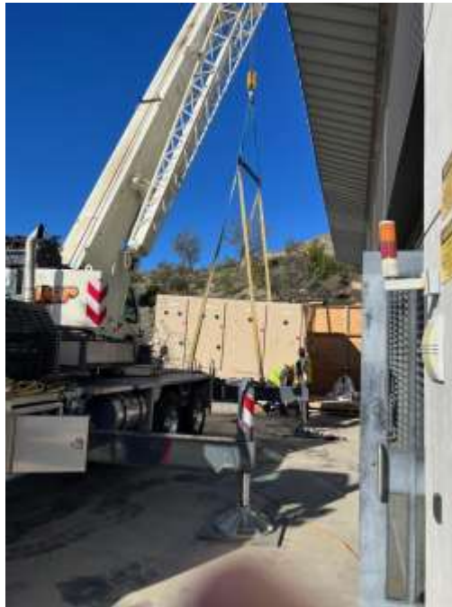
Jensen Ozone PSUs Replacement—Unloading power supply unit
