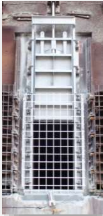
New Gate No. 12 installed
