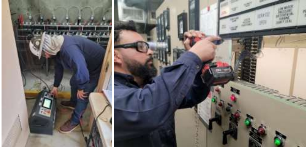
Staff performing battery testing (left) and data logger replacement (right) at Lake Matthews HEP
