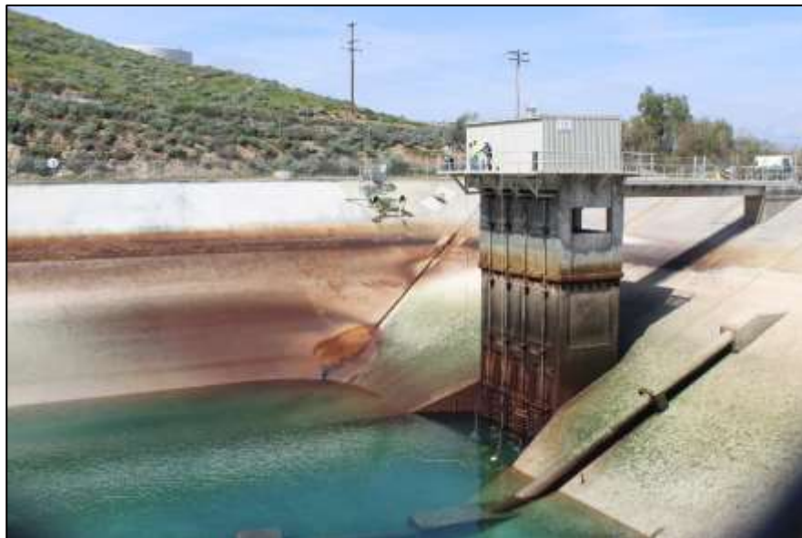
The forebay outlet tower during the dewatering process at Lake Mathews
