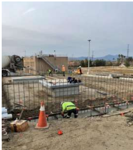
Mills Electrical Upgrade—RPU Switchyard—Concrete Placement near electrical vault
