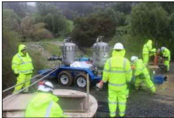
Staff setting up for dewatering on the Santiago Lateral
