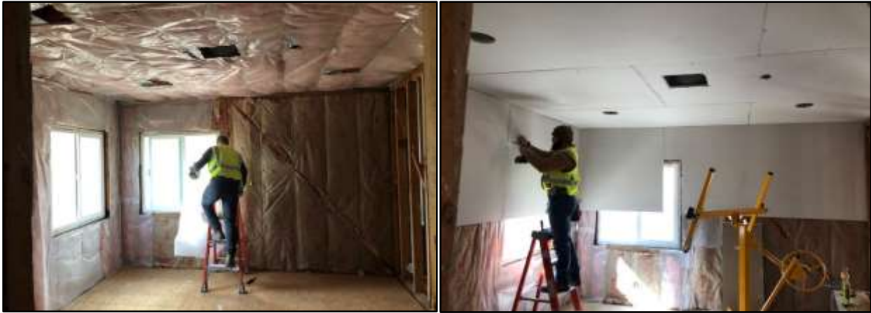
Insulation and Drywall Installed at Iron Mountain Wellness Center
