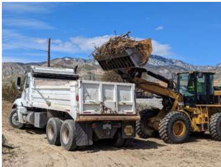
Staff loading a dump truck with vegetation from along the CRA
