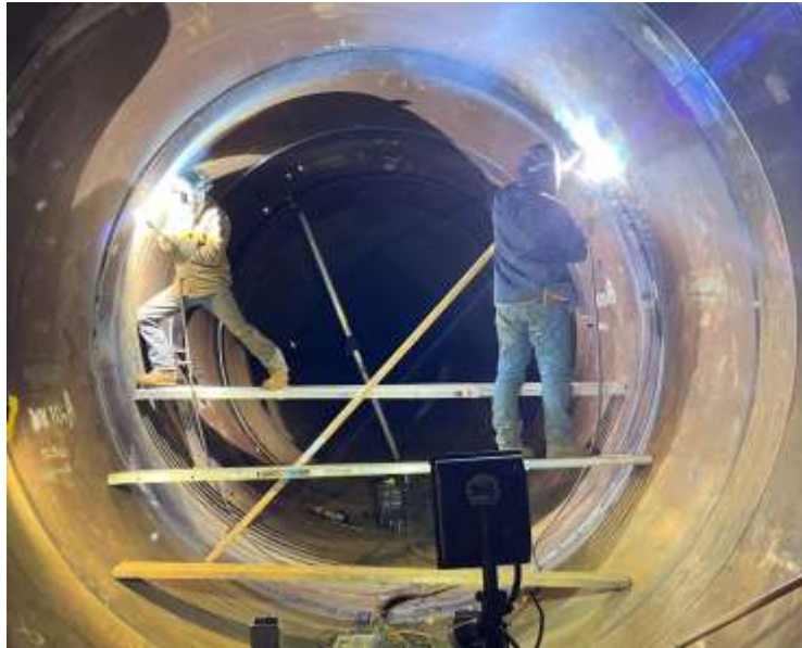
Etiwanda Pipeline Relining—Welding steel pipe Buttstraps
