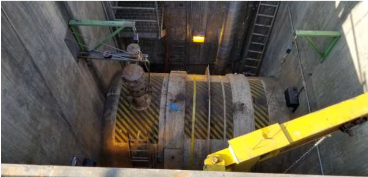
Large roll-out section installed at Santa Ana Valley Pipeline
