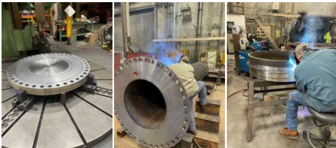
Machining of bulkhead flange (left) and fabrication of lower bulkhead segments (middle and right) for Red Mountain PCS
