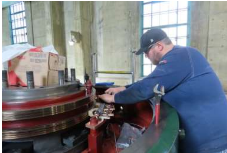
Staff replacing a carbon ring brush at Hinds pumping plant
