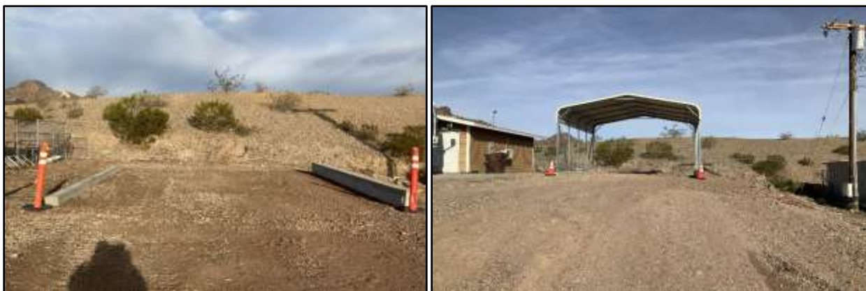
Before and After Carport Installation at House 48-G
