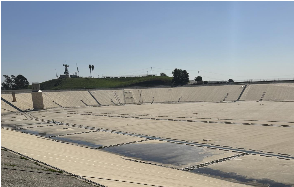
The existing reservoir floating cover overview at Garvey Reservoir
