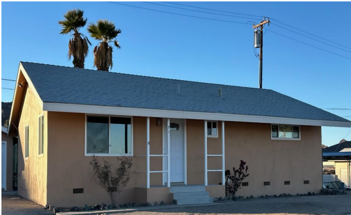
Existing employee single-family house – Eagle Mountain Pumping Plant
