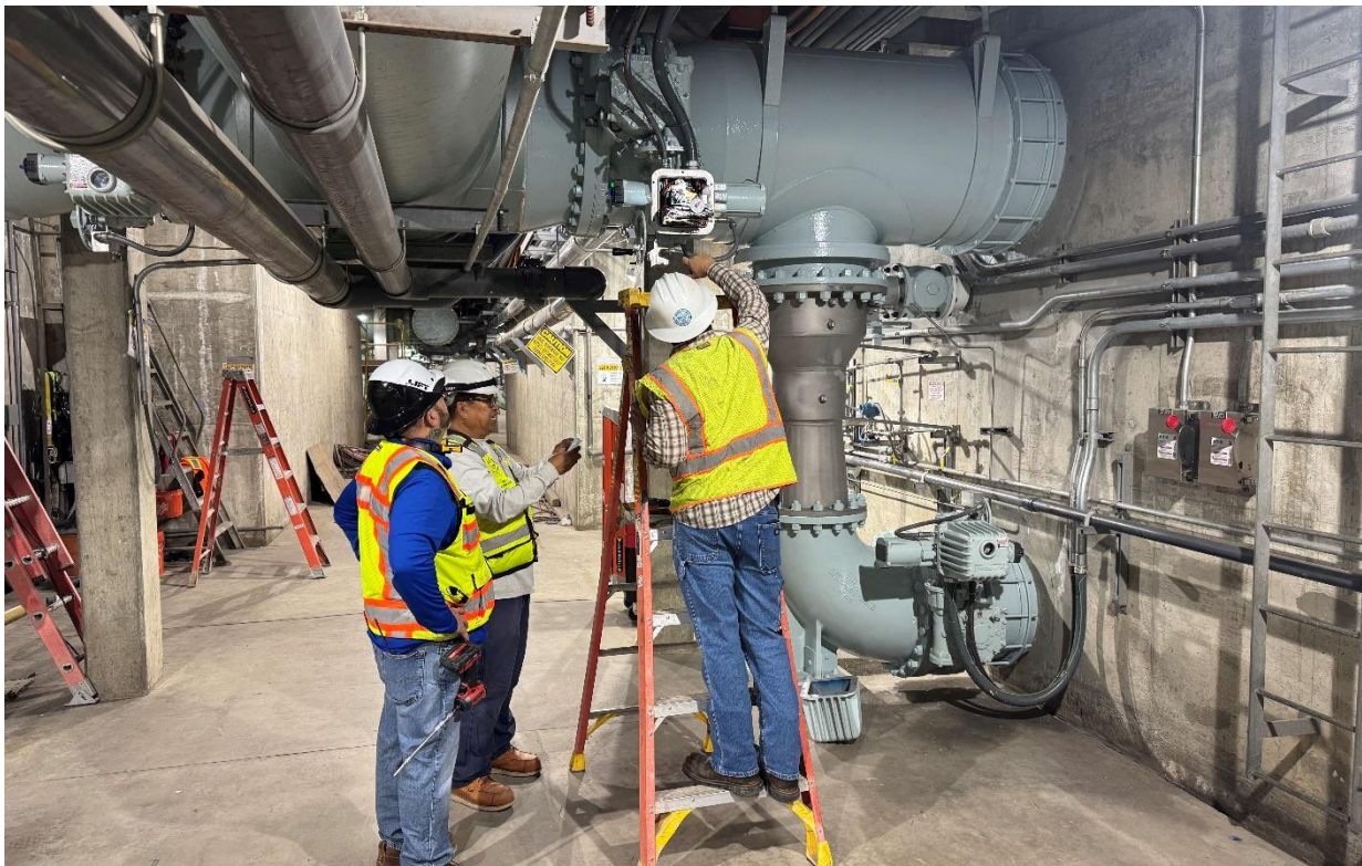
Conducting valve actuator functional testing under the Filter Building No. 2
