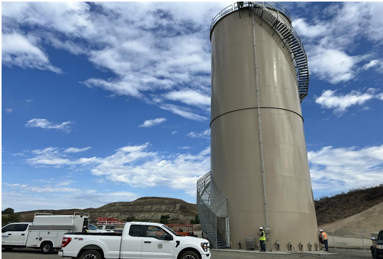
Inspecting the surge tank exterior
