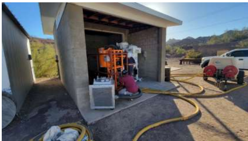
Staff setting up and testing abrasive blasting equipment for coating work
