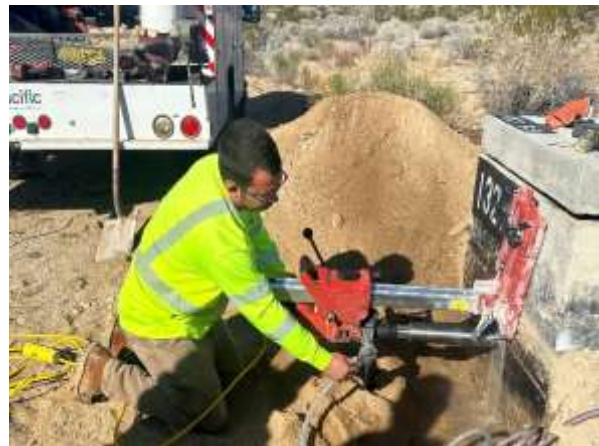
Staff excavating (left) and drilling into a structure (right) to place a level transducer for CRA monitoring
