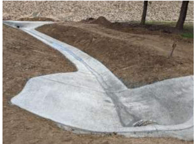
Staff removing old concrete (left) and a newly completed concrete V-ditch with apron (right) at the Skinner Dam
