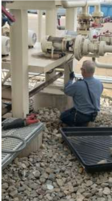
Staff replacing a 230kV transformer oil pump at a Desert facility
