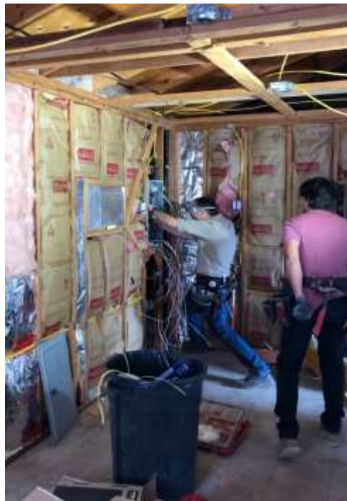
Staff performing electrical panel upgrades at Desert housing structure
