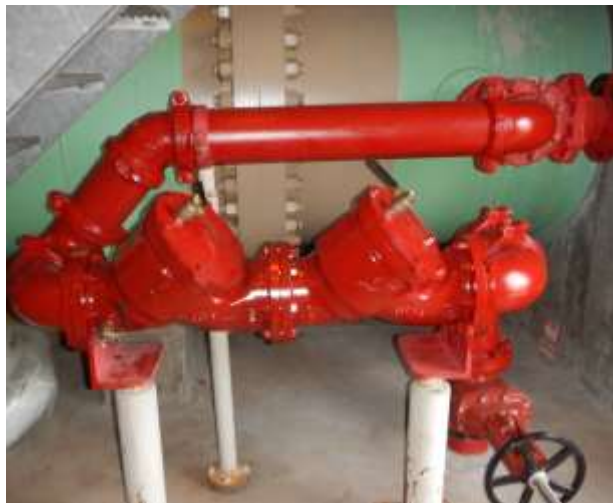
OC-88 Fire Sprinkler—New backflow preventer and piping
