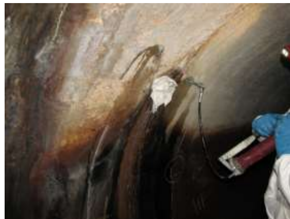
Staff performing hydrophilic injection repairs inside the Rainbow Tunnel
