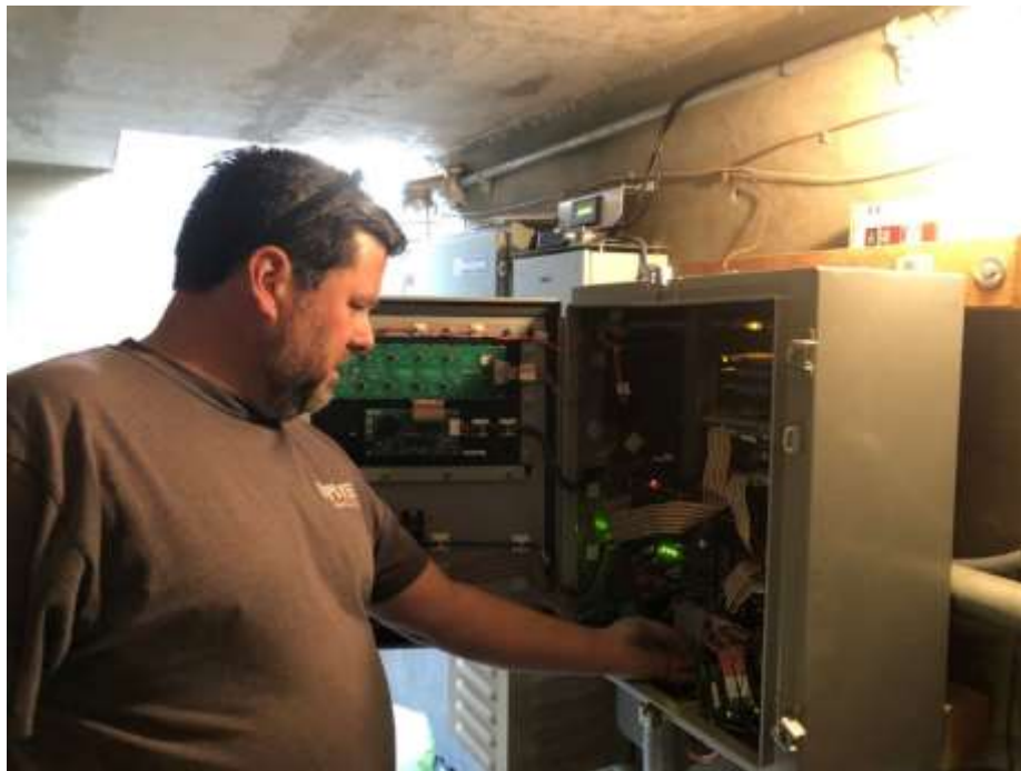
Staff repairing a flow meter at service connection
