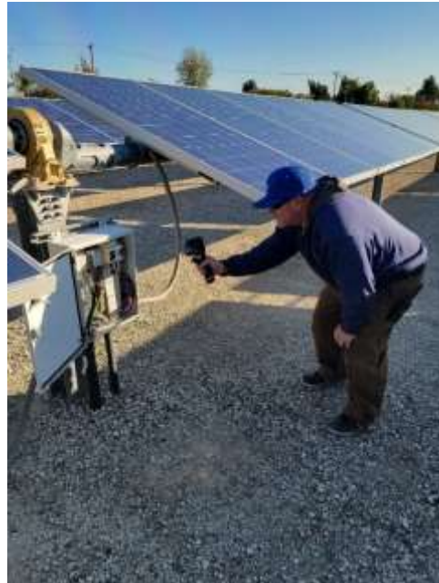
Staff recording combiner box post-repair temperatures at the Weymouth plant
