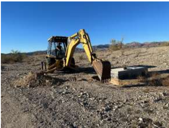
Staff excavating (left) and drilling into a structure (right) to place a level transducer for CRA monitoring
