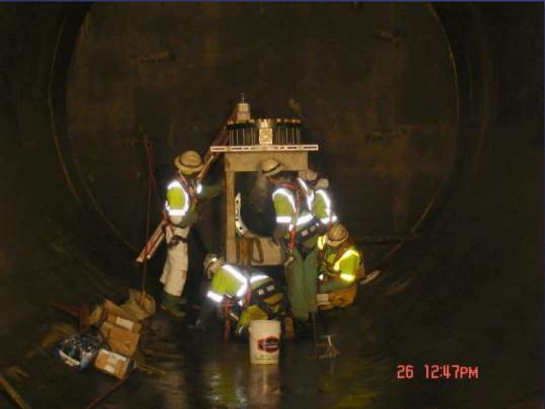
Installing Butterfly Valve in the Foothill Feeder
