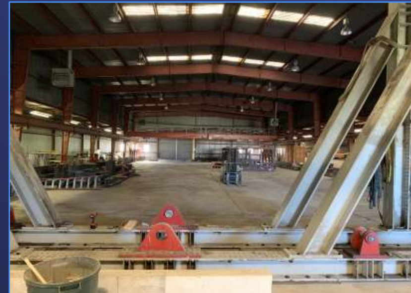
Pre-Phase 1 CSI Building
