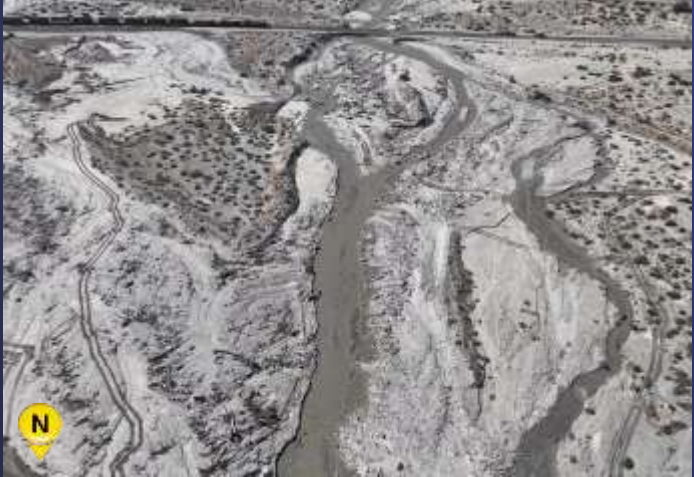
Damage to Main Channel
