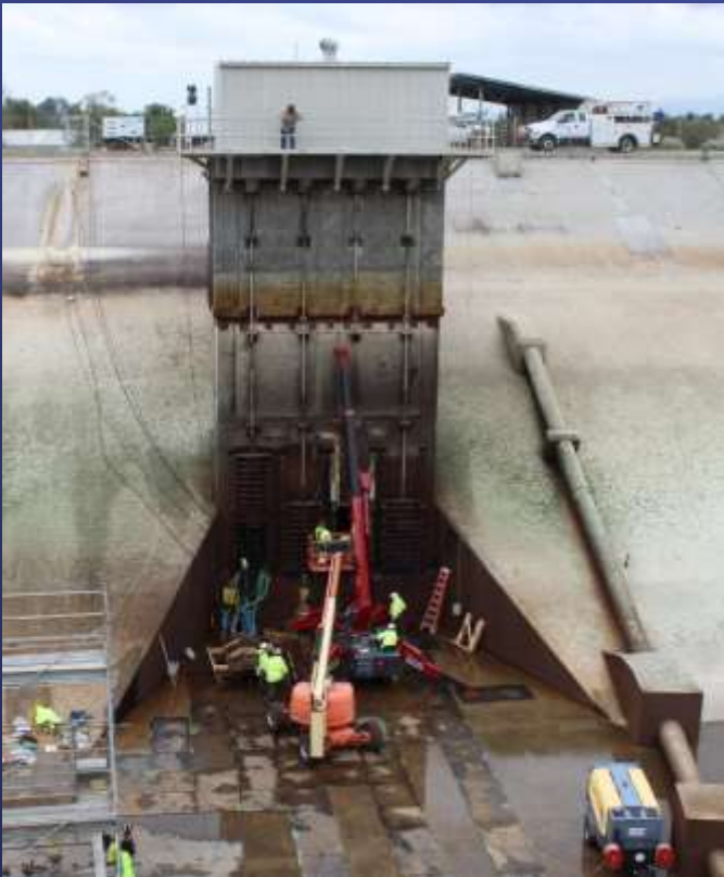
Installing Lake Mathews Forebay Gate
