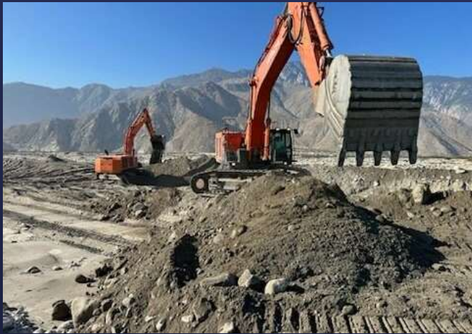
Metropolitan staff repairing Main Channel
