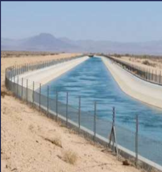
Colorado River Aqueduct August 30
