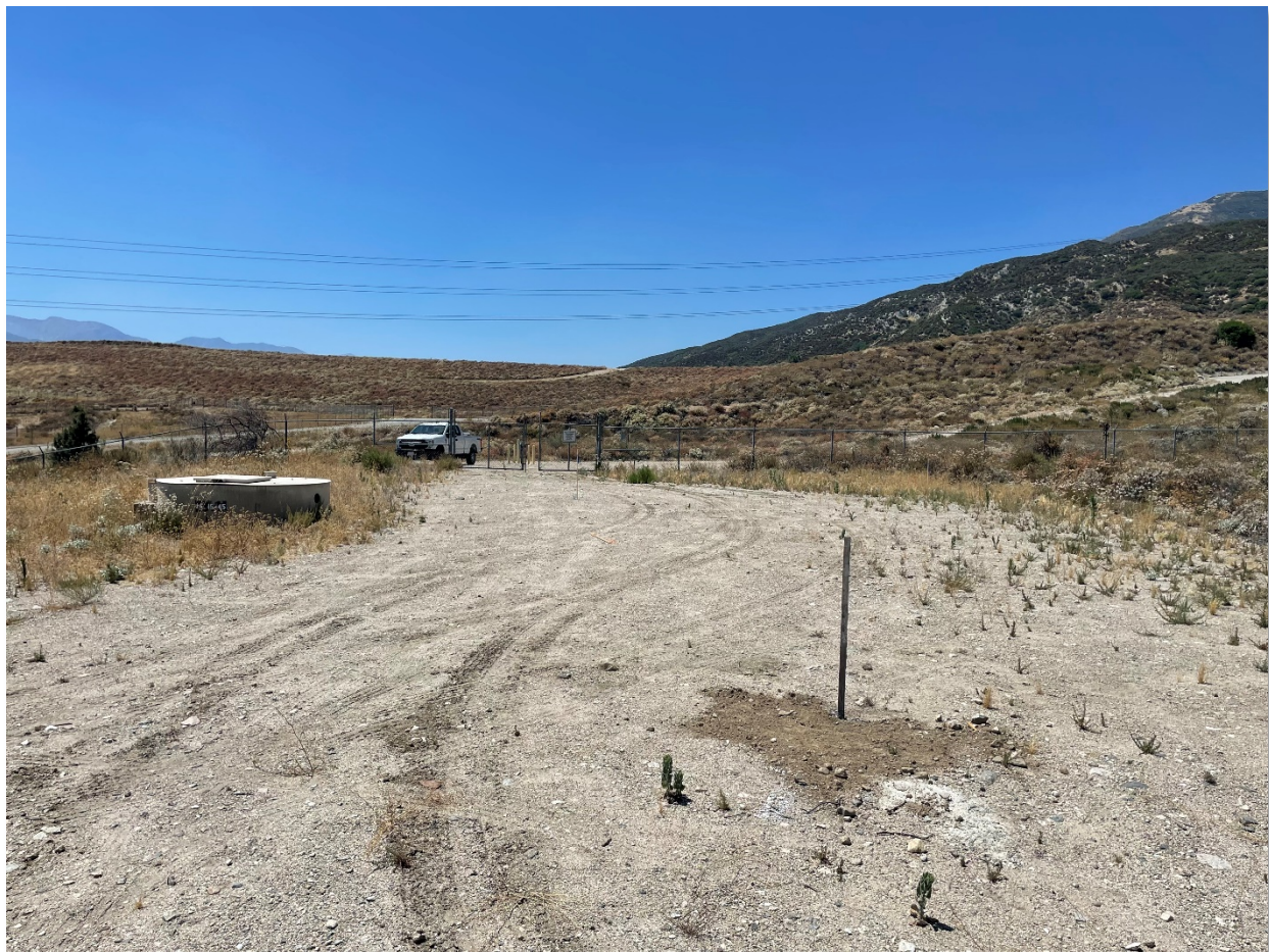
Inland Feeder/Rialto Pipeline Intertie project site looking in the northwesterly direction towards DWR’s Devil Canyon Afterbay No. 2 Embankment
