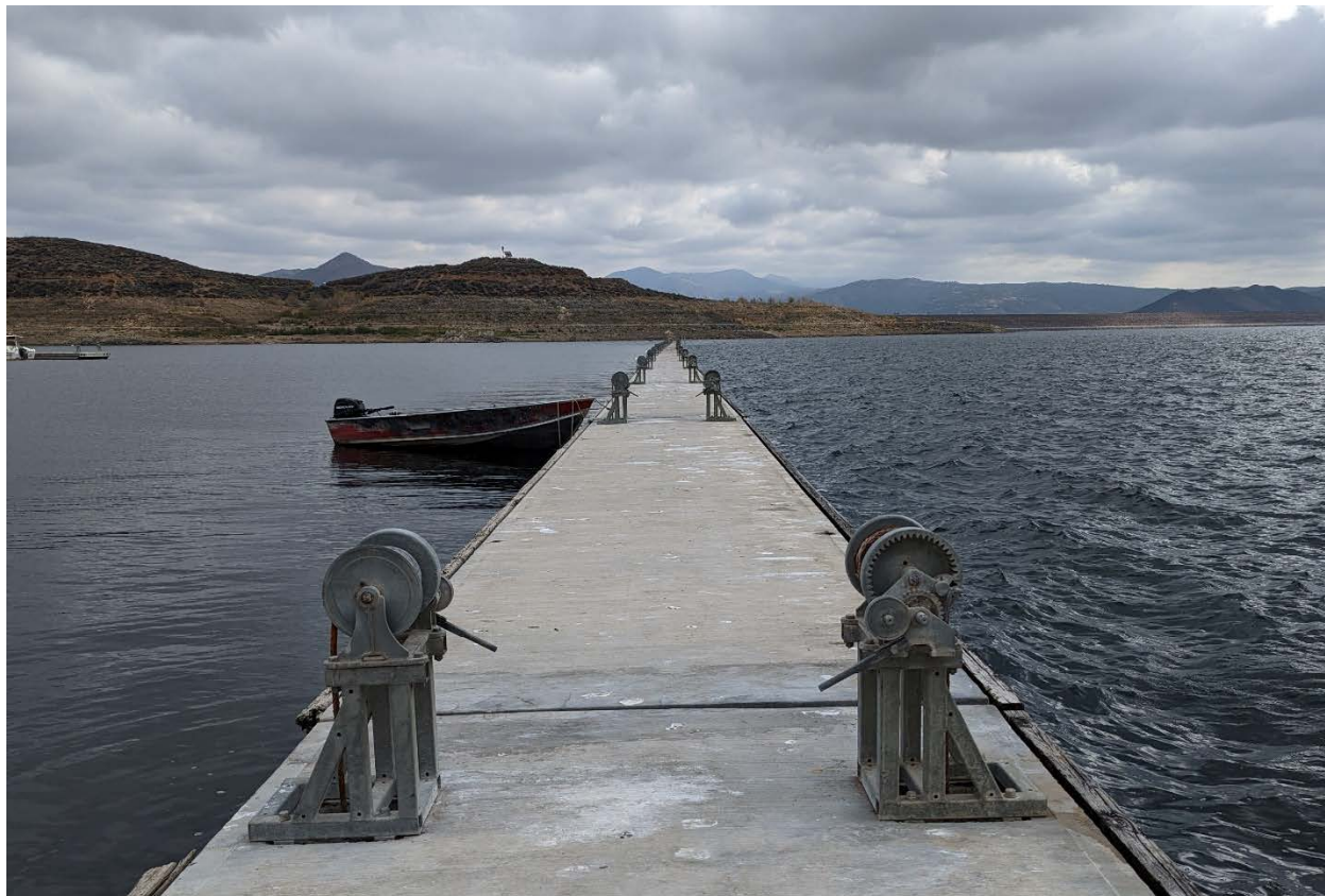
Existing floating wave attenuator at Diamond Valley Lake: Looking from West to East
