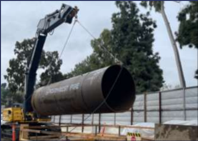
Second Lower Feeder PCCP Relining
