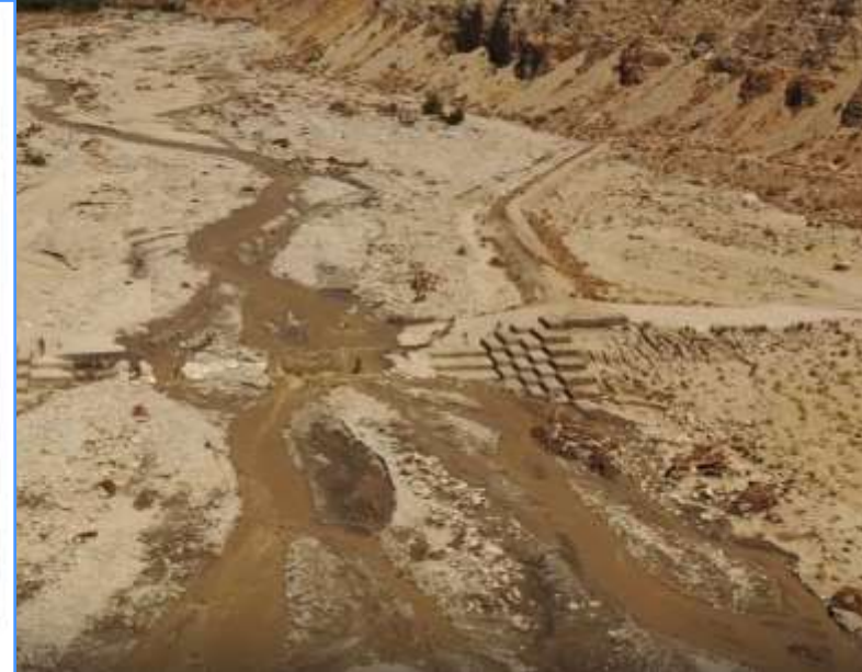
2023 view of siphon post-storm event
