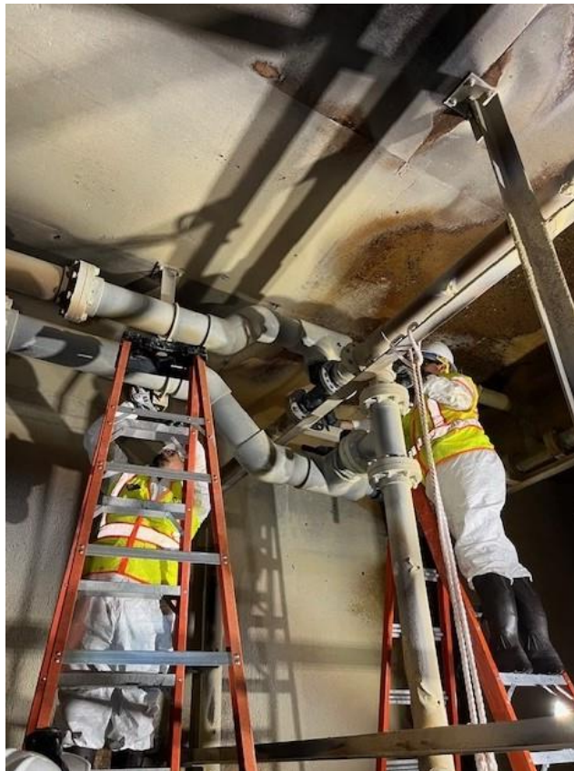
Staff repairing chlorine diffuser inside the combined filter effluent channel at the Diemer plant
