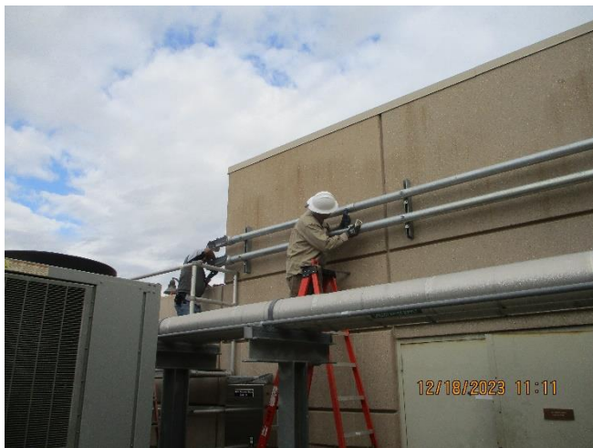
Staff installing new electrical (left) and completed conduit installation (right) at the Water Quality Laboratory
