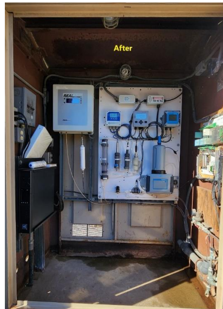
Old (left) and new (right) water quality panel at the Palos Verdes Reservoir
