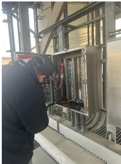
Staff terminating wiring and securing control panel at chemical tank farms at the Weymouth plant
