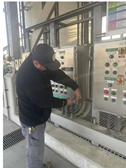
Staff terminating wiring and securing control panel at chemical tank farms at the Weymouth plant
