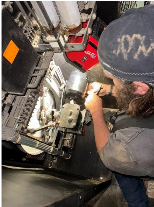
Staff installing a DC rheostat on a CRA pump motor
