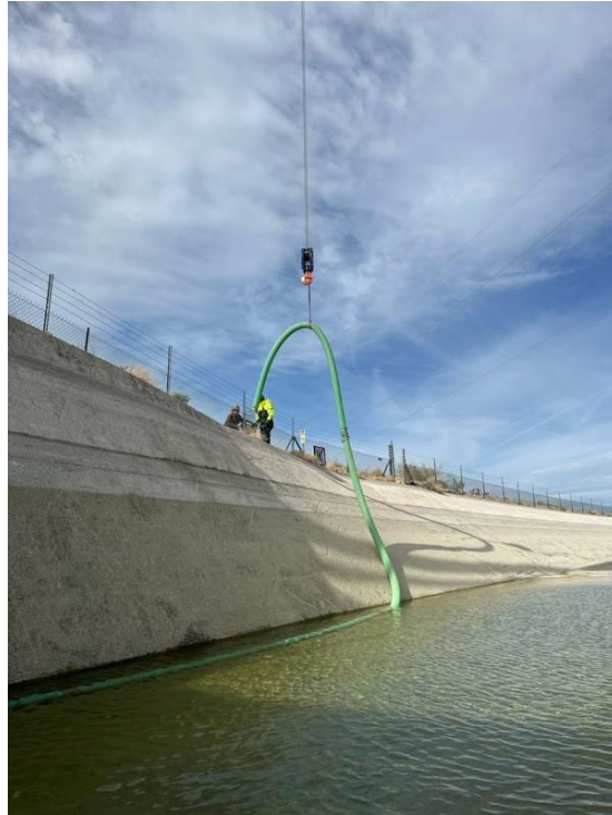
Staff dewatering the CRA using portable pumps
