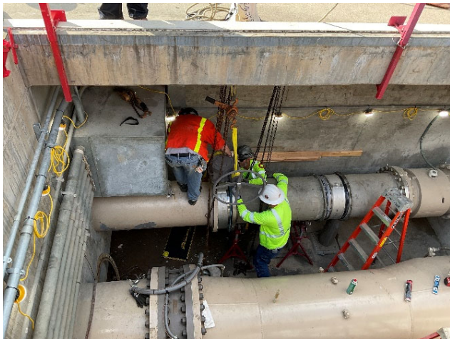
Staff installing replacement valve (left) and hoisting valve with truck crane (right) at the Jensen plant
