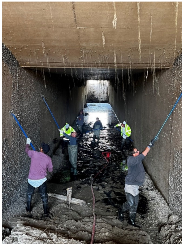
Staff manually scraping debris in the low siphons of the San Diego Canal
