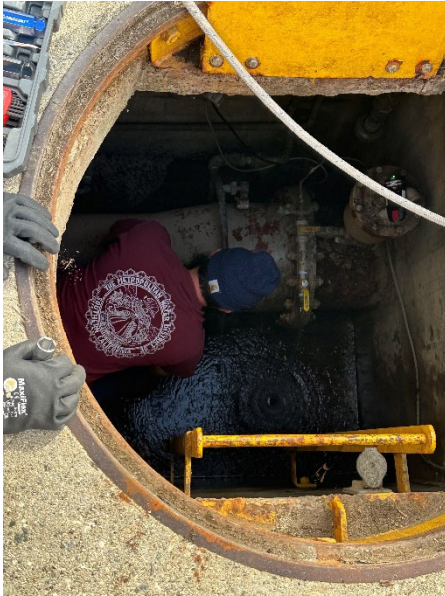
Staff replacing Victaulic meter port
