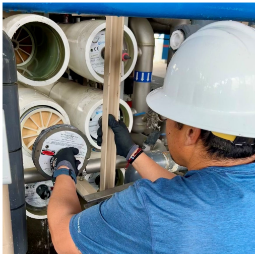
Staff installing a new RO membrane at the demonstration plant following an extraction for analysis
