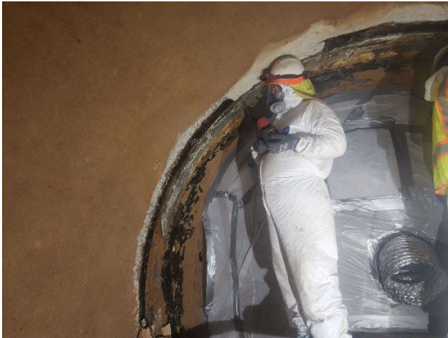
Staff repairing transition joint at Eagle Mountain pumping plant
