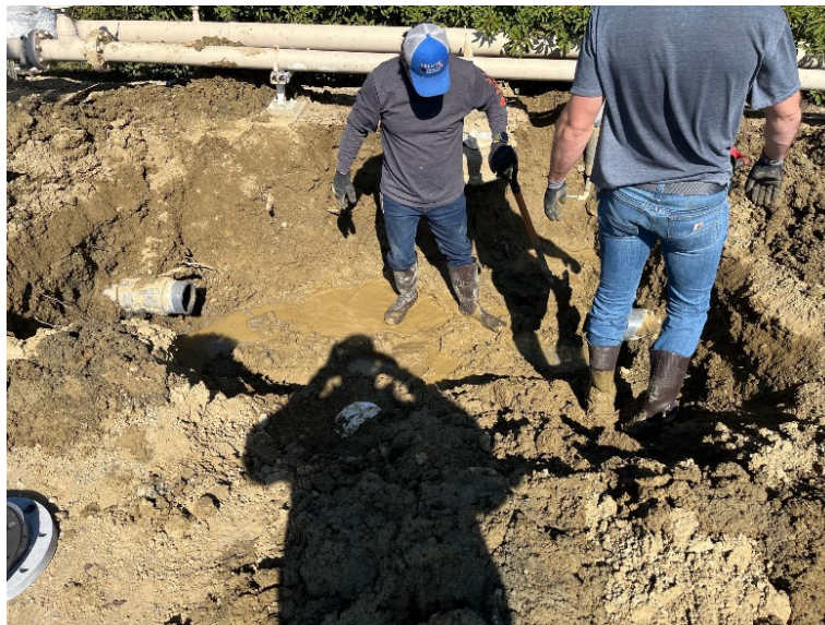
Staff repairing a broken water line at the Diemer plant
