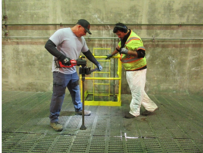
Staff exercising a plug valve during routine preventive maintenance at Venice PCS
