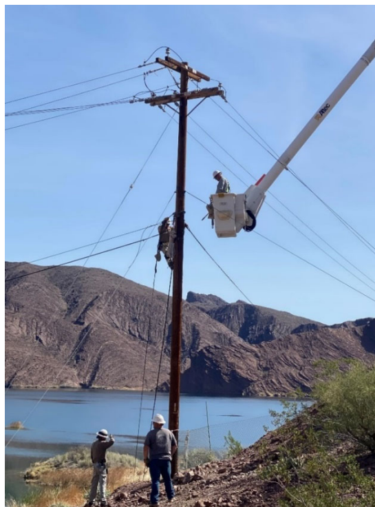
Staff isolating a 2300V circuit at Copper Basin
