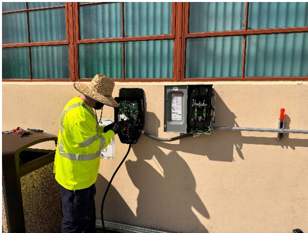
Staff terminating conductors (left) and installing electrical equipment (right)
