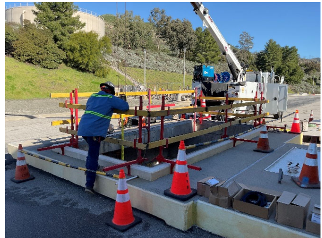
Staff installing replacement valve (left) and hoisting valve with truck crane (right) at the Jensen plant
