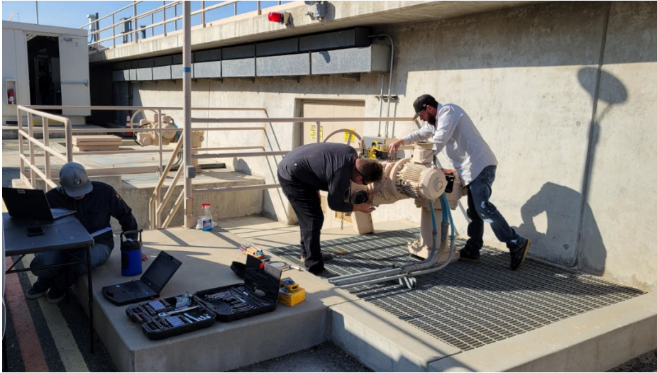
Staff troubleshooting contactor inlet butterfly valve (left) and new turbidity meters installed in the cross tunnel (right) at the Mills plant
