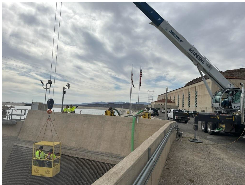
Staff removing trash racks at Eagle Mountain pumping plant
