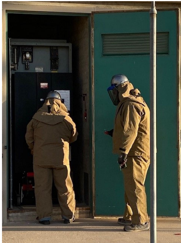
Staff racking out a 6.9kV circuit breaker at Gene pumping plant
