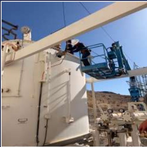
Hinds Pumping Plant Transformer Repair
