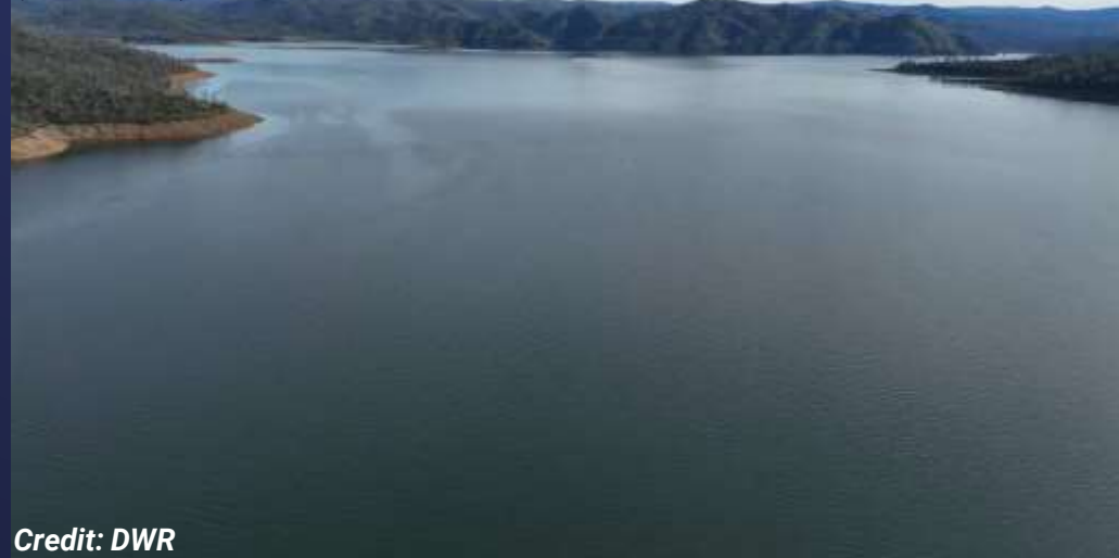
Lake Oroville, Banks Pumping Plant, California Aqueduct (March 2024)
