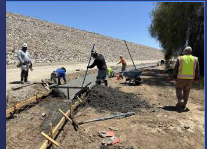
V-Ditch Concrete Placement
