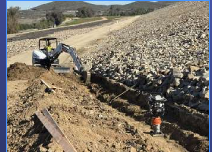
Excavation for new V-ditch
