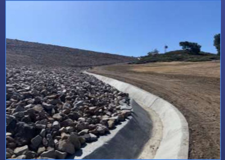
V-Ditch near Left Abutment Looking Upstream
