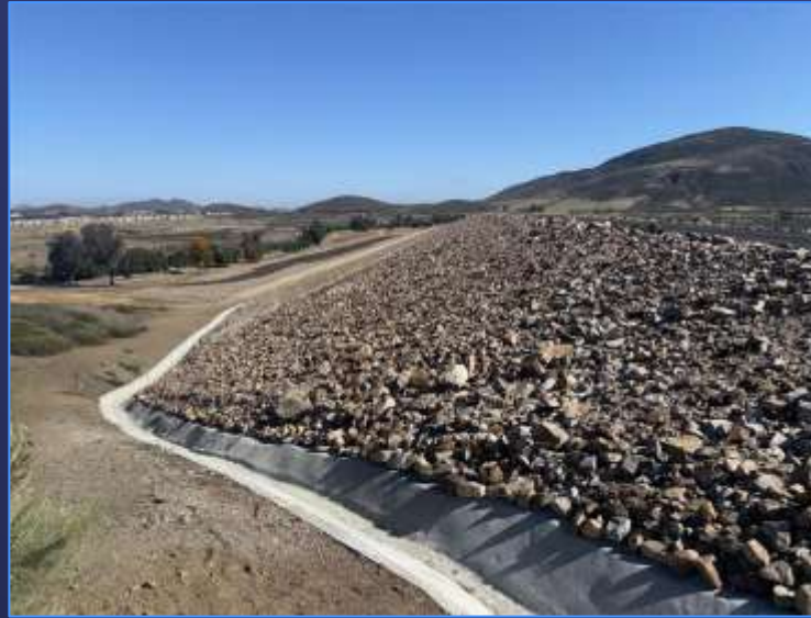
V-Ditch near Left Abutment Looking Downstream
