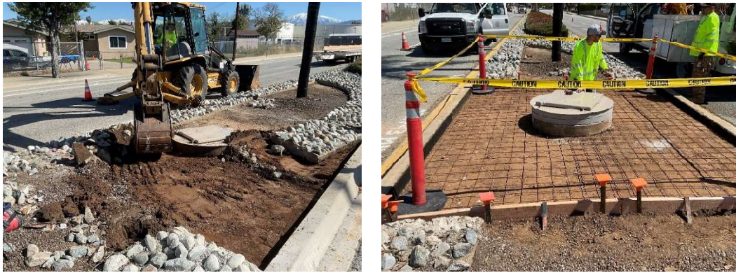
Staff excavating concrete slab area (left) and reinforcing wire installation (right) to enhance safe access at a Middle Feeder structure
