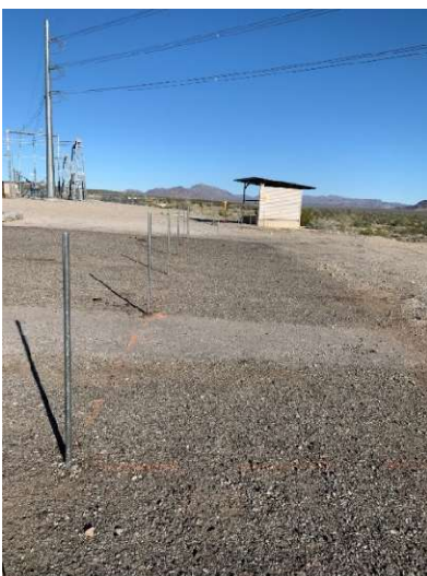
Temporary fencing to protect desert tortoise and other animals from entering construction zone at Hinds pumping plant
