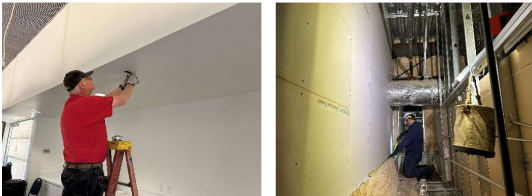
Staff installing a new cut-in box (left) and electrical conduit (right)
