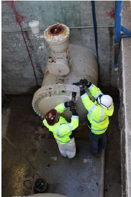
Staff removing flanges to provide access for contractors to complete relining work for the AMP
