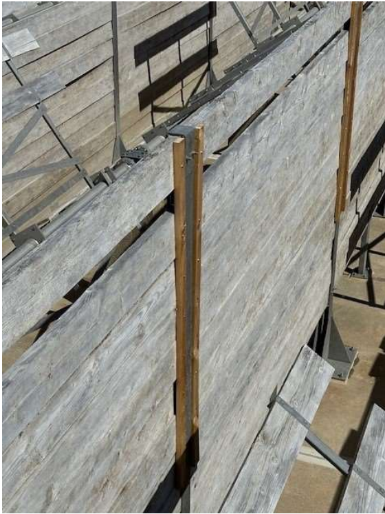
Staff securing baffle boards inside the sedimentation basin at the Diemer plant
