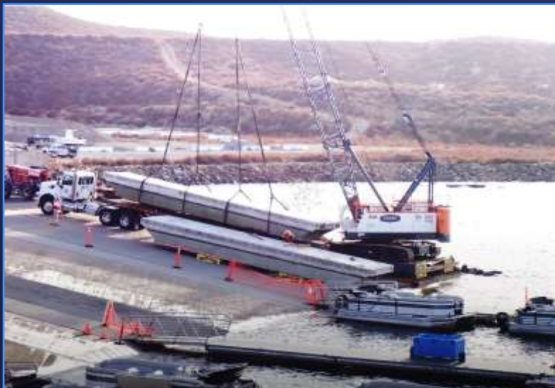
Courtesy Dock Segment Removal
