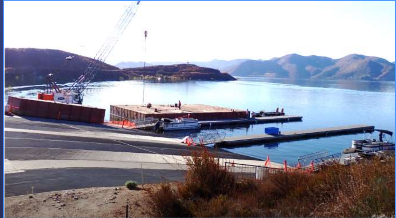
Assembling Modular Flexi-Float Barge System
