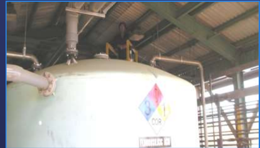
Tank Farm Roof Clearance
