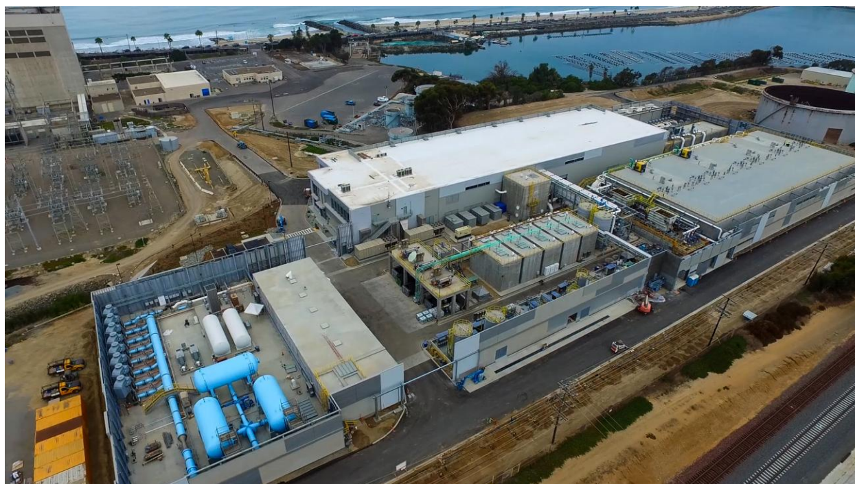
Figure 6.4 Carlsbad Seawater Desalination Plant (Courtesy of Dudek)
