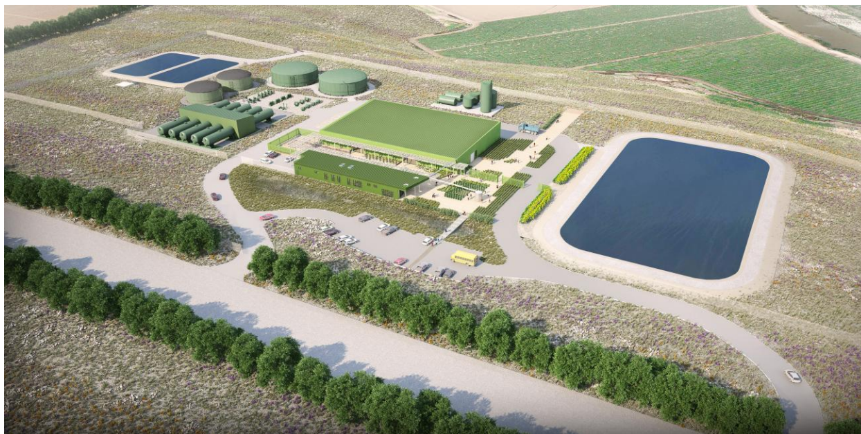
Figure 6.3 Monterey Seawater Desalination Plant
