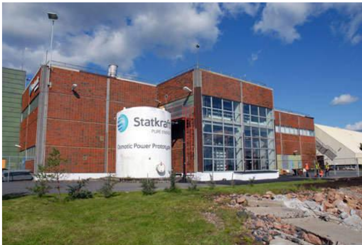
Figure 3.14 Prototype PRO Facility in Tofte, Norway (Courtesy of Statkraft)
