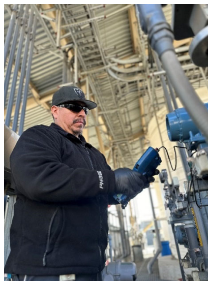
Staff calibrating alum flow meter (left) and staff calibrating polymer flow meter (right)
