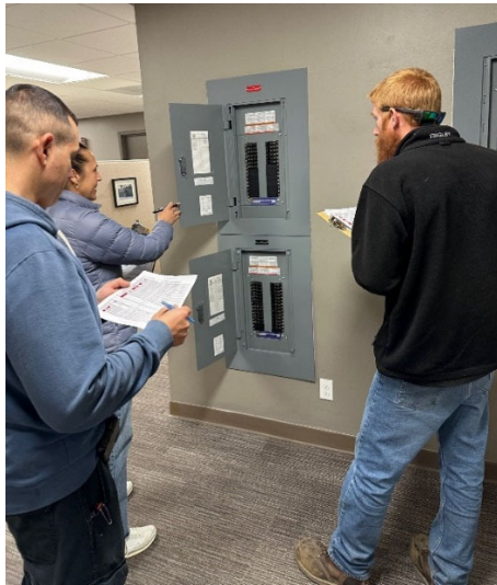
Staff verifying labels on the electrical breaker panels
