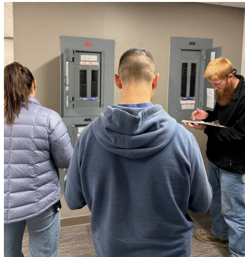
Staff verifying labels on the electrical breaker panels
