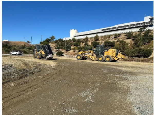
Motor grader performing site grading for construction of Helicopter Hydrant Facility.
