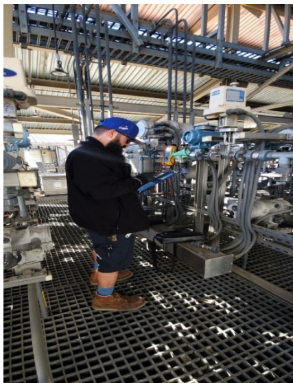
Staff calibrating alum flow meter (left) and staff calibrating polymer flow meter (right)
