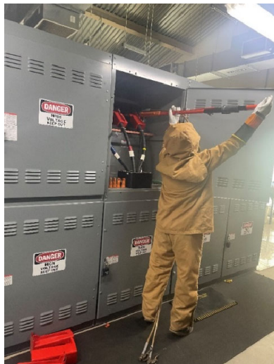
Electrician grounding conductors before work (left) and electricians preparing high voltage termination (right)
