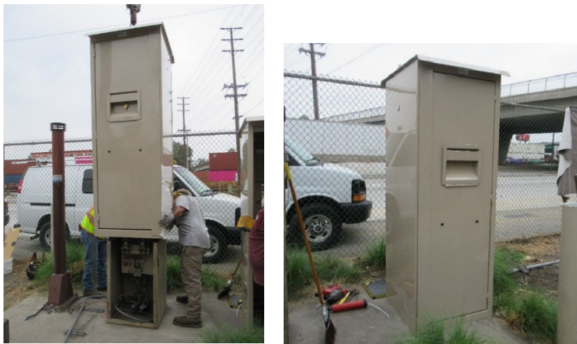
Staff installing two high-security meter cabinets at service connection LA-16
