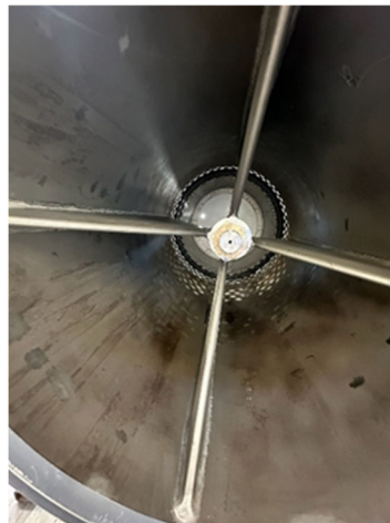
Installation of valve shaft (left), installation of valve shaft nut (middle) and installed new stem nut cover (right)
