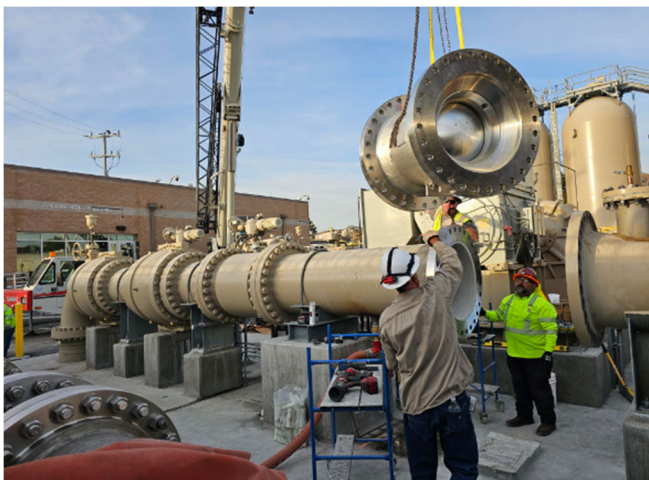
Staff hoisting check valve into place (left) and constructing new pipe support (right)
