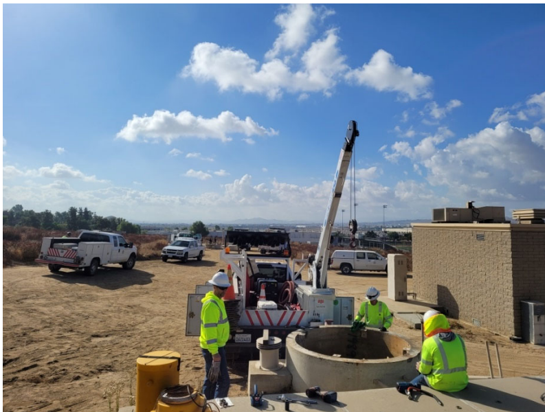
Staff providing top support at the Perris Bypass Pipeline shutdown
