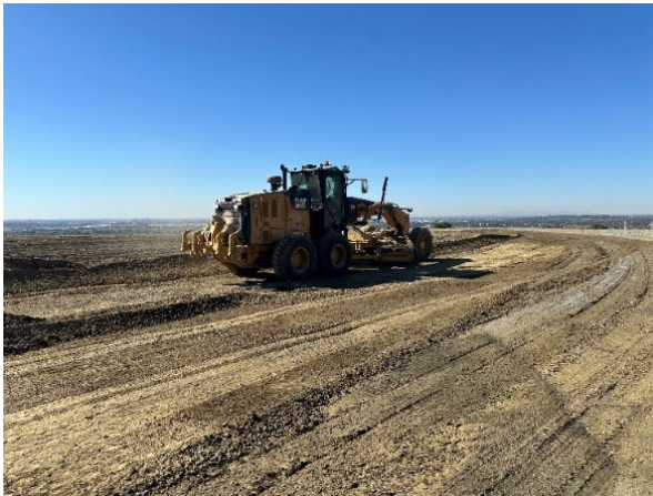
Motor grader performing site grading for construction of Helicopter Hydrant Facility.
