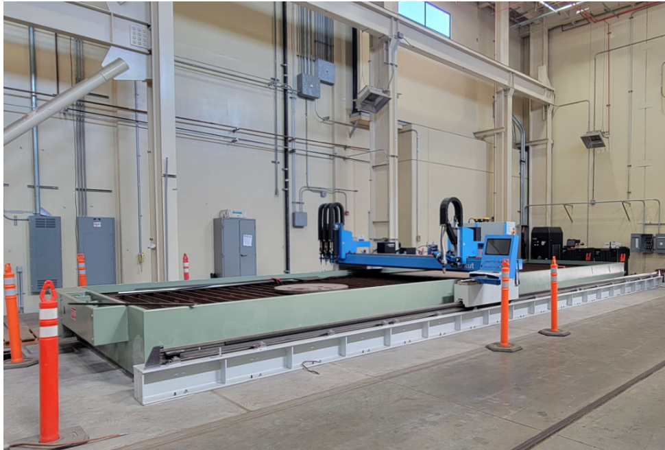
La Verne Shop Improvements—New Plasma cutter and water table
