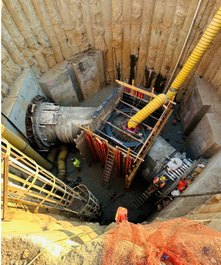
Perris Valley Pipeline—Preparation of Shaft 3 Accessway Encasement
