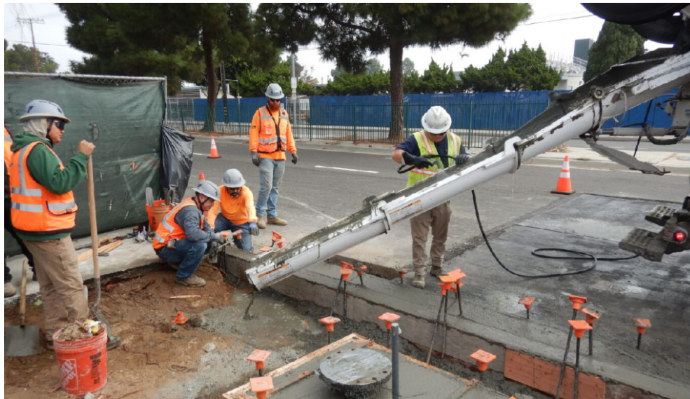
Second Lower Feeder Reach 3B—AR/VV-Concrete Placement
