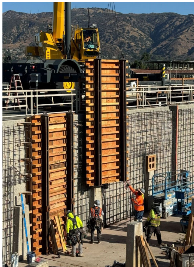
Weymouth Basins 5–8 and Filter Building No. 2 Rehabilitation—Setting concrete formwork at Basin 5
