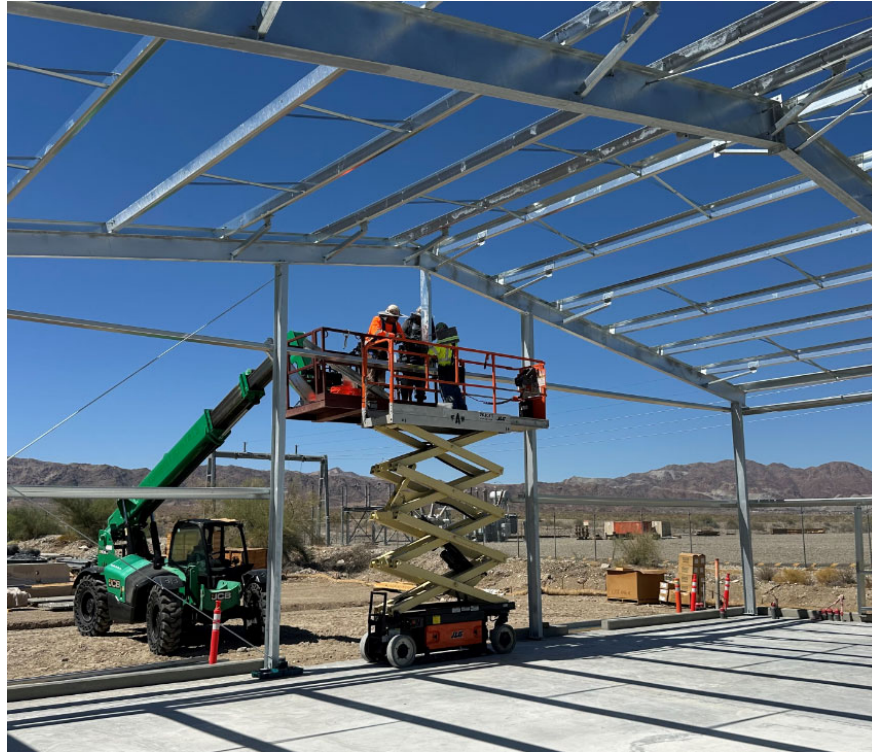
CRA Storage Buildings – Eagle Mountain Pumping Plant - installing framing
