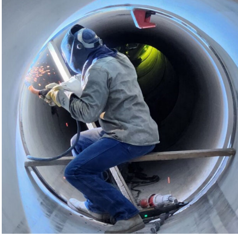
Allen-McColloch Pipeline (AMP) Urgent Relining 2024—Welding of 60-inch Diameter Steel Liners
