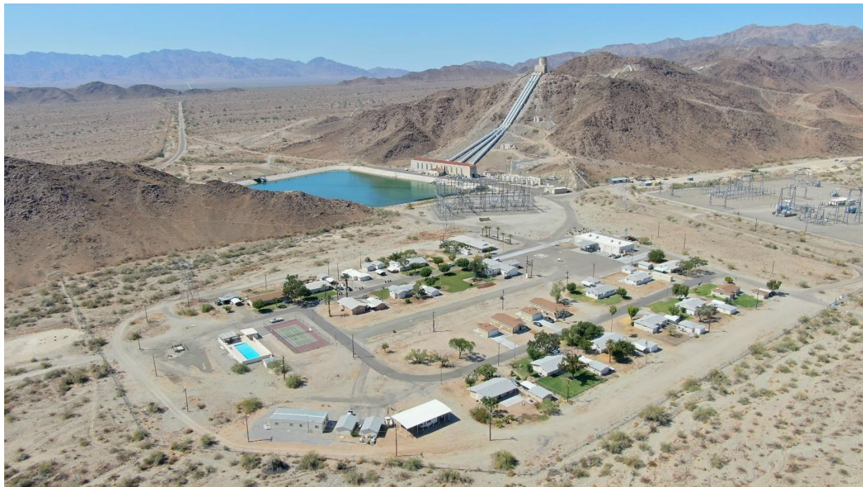
Existing village site of future improvements – Eagle Mountain Pumping Plant
