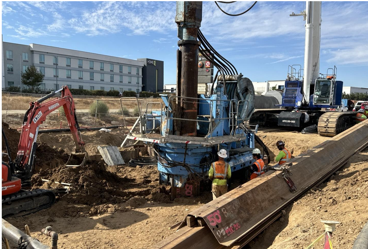
Sheet piling installation at the northern tie-in to Perris Valley Pipeline
