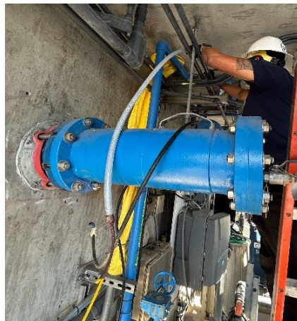
Installation of a new chemical line for the carbon dosing system at the PWSC Napolitano Center
