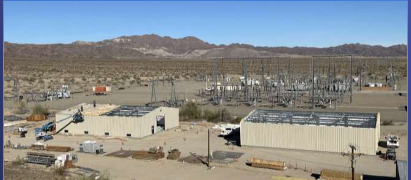
Eagle Mountain Buildings
