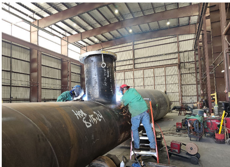
Allen-McColloch Pipeline (AMP) Urgent Relining— Welding accessway on 48-inch access pipe
