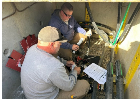
Electrician grounding conductors before work (left) and electricians preparing high voltage termination (right)
