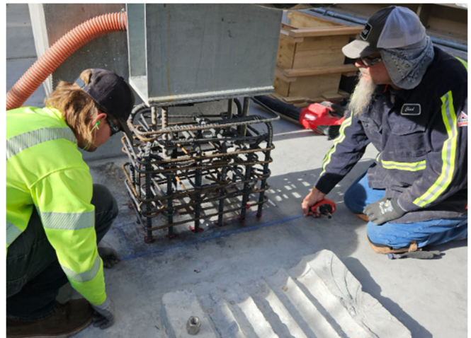
Staff hoisting check valve into place (left) and constructing new pipe support (right)
