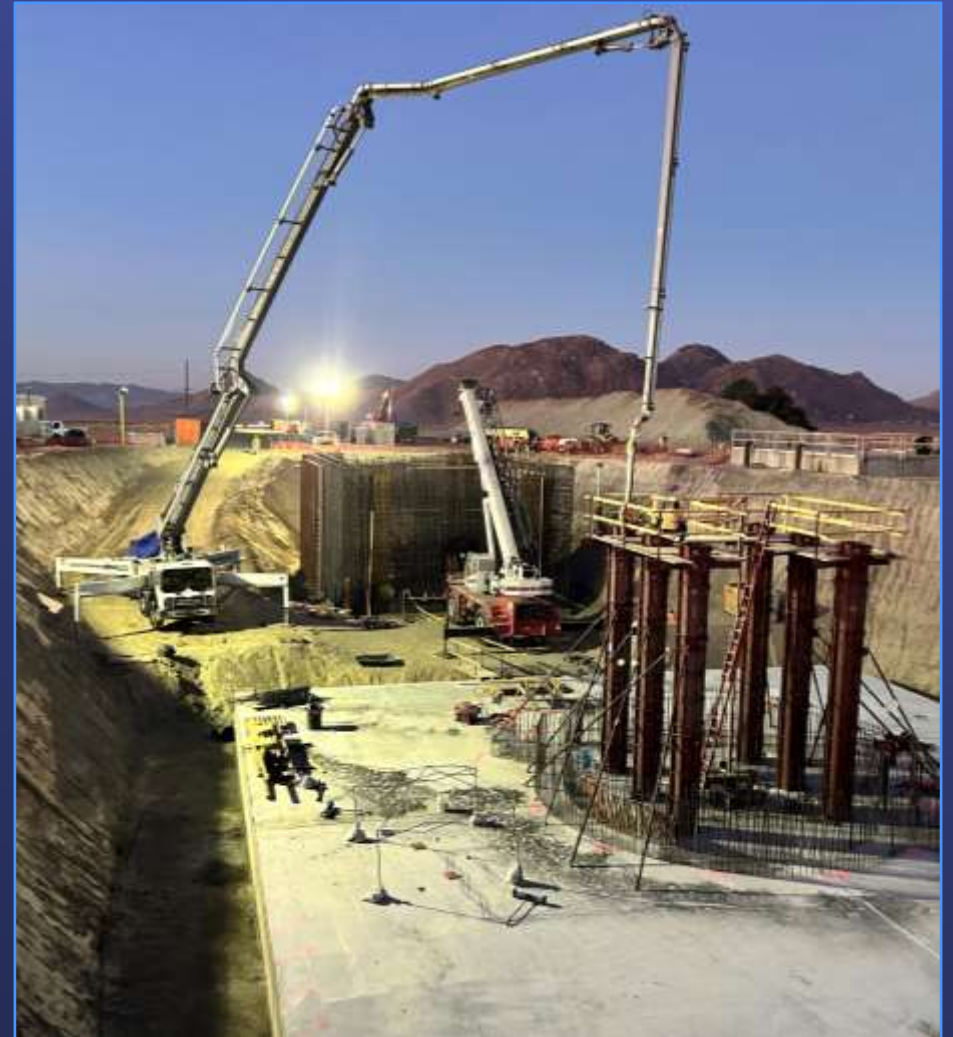
Contractor Placing Concrete for Surge Tank Footings
