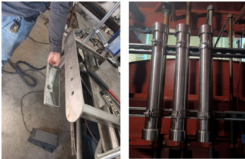
Lubrication oil sample tap bracket (left) and lubrication oil sample manifold (right)
