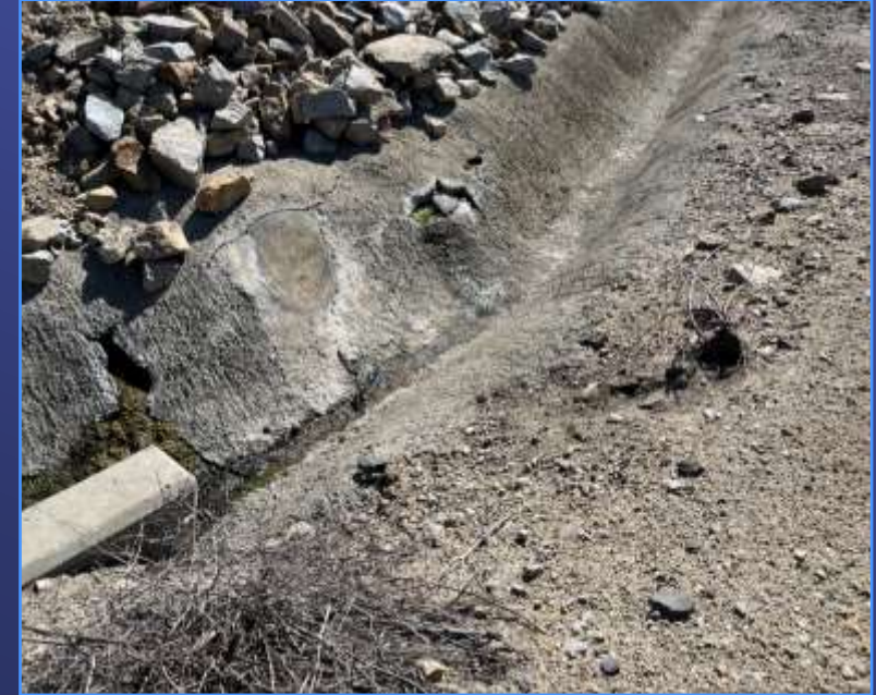
Existing Drainage Control Ditch
