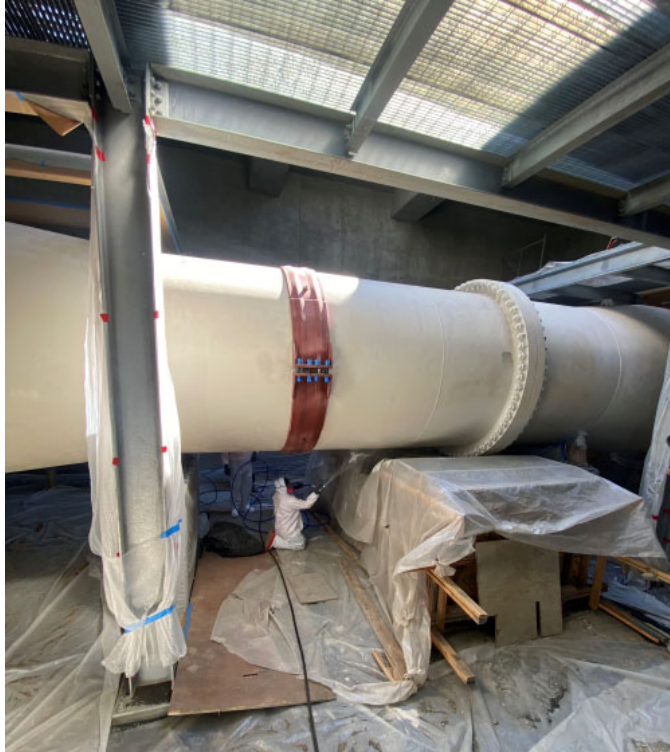
Wadsworth Bypass—Wadsworth coating 96-inch pipe within valve vault
