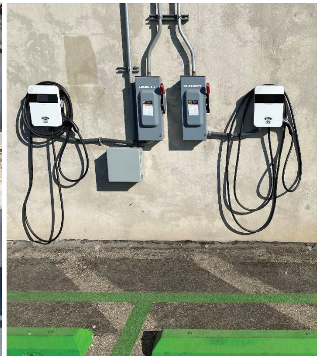
Level 3 EV charger (left) and Level 2 EV chargers (right) at Weymouth Water Treatment Plant
