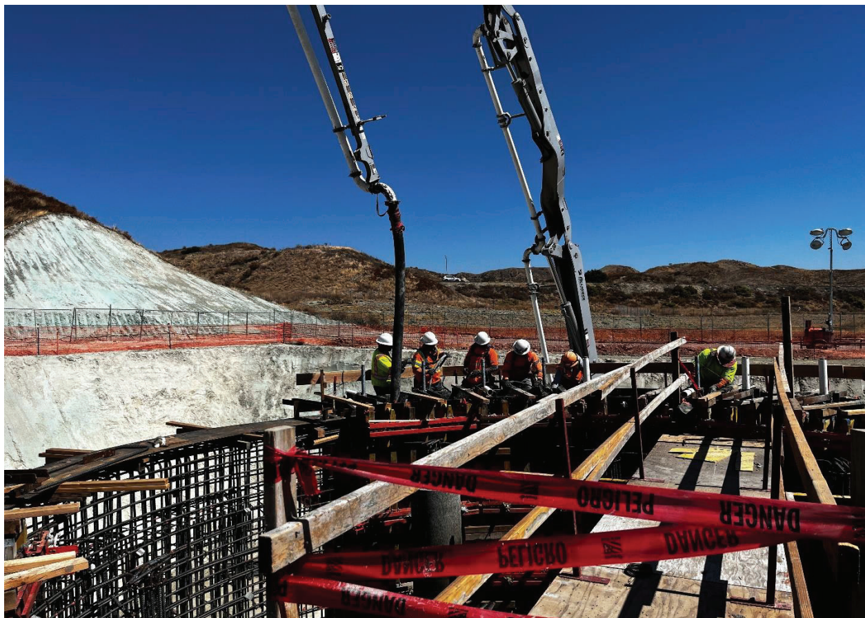
Contractor placing concrete for the surge tank wall
