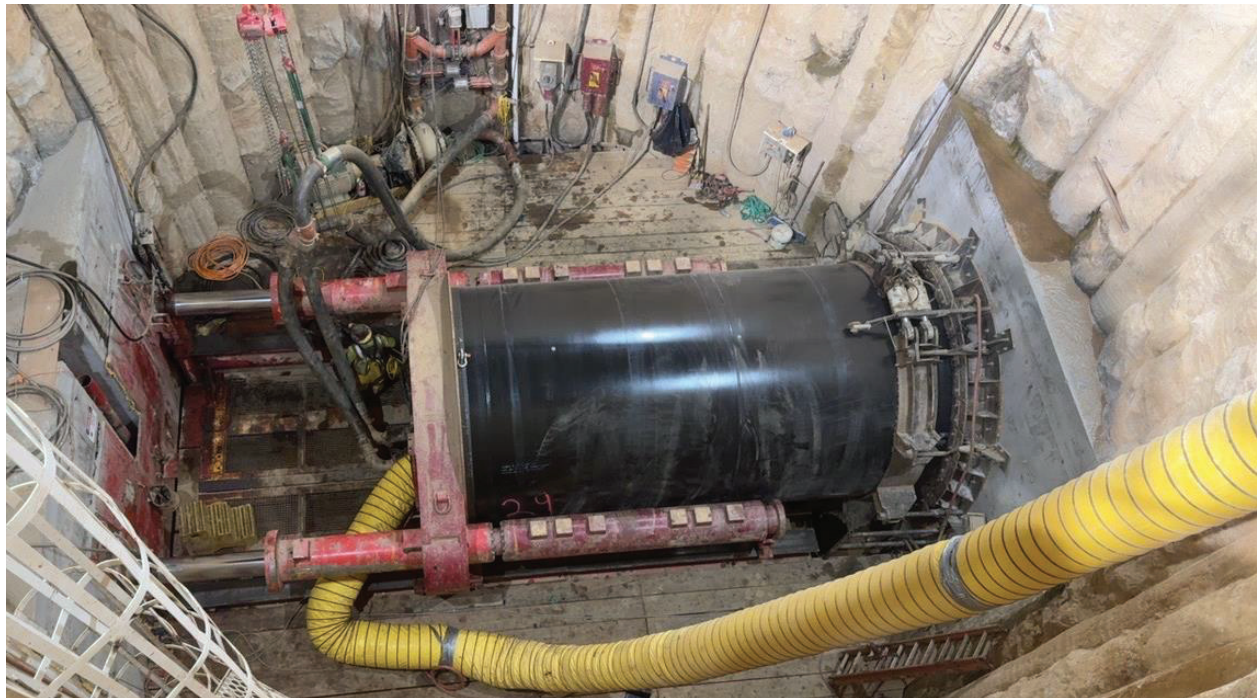
Secant pile shaft during installation of 120-inch diameter casing at Shaft No. 1 to the northern tie-in of Perris Valley Pipeline
