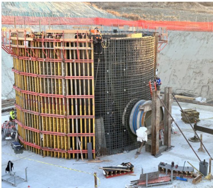
Inland Feeder-Badlands Tunnel Surge Protection—surge tank wall formwork
