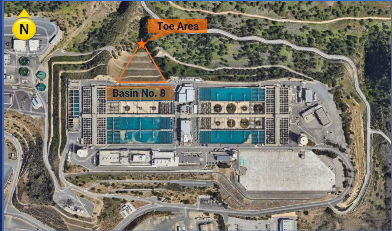
Overview of Diemer Plant
