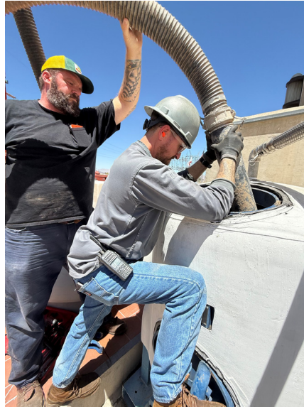
Staff replacing the GAC media for the domestic water system at Eagle Mountain pump plant
