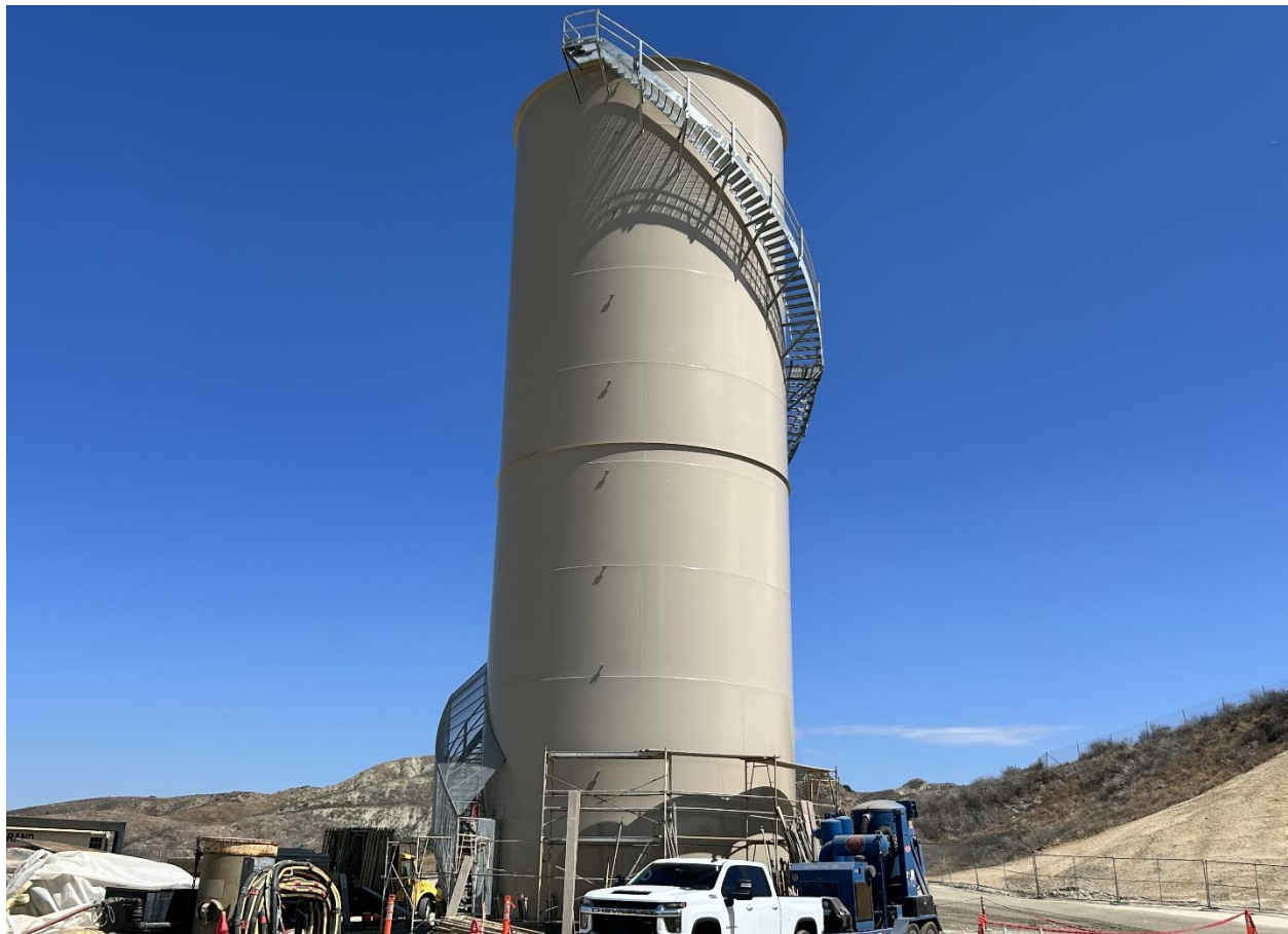
Applying exterior coating to the surge tank
