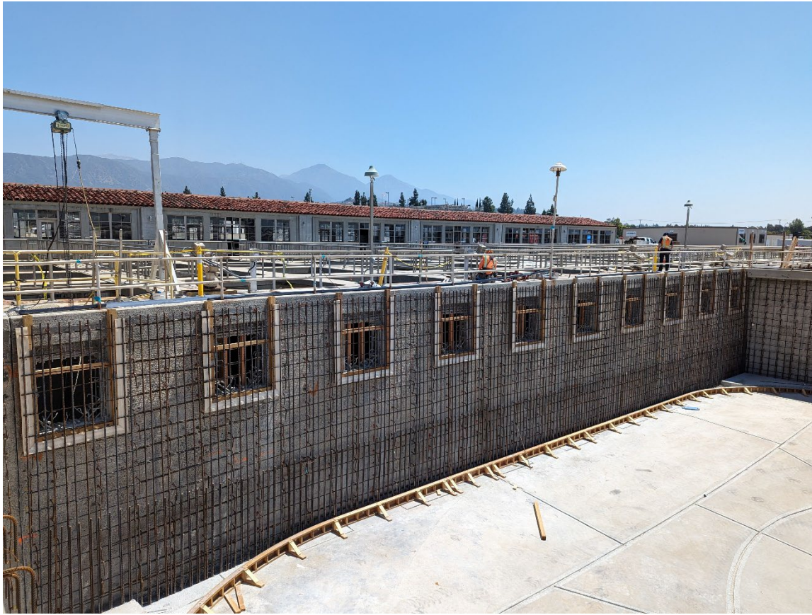
Figure 4-1: Seismic Reinforcement of Weymouth Basin 7
