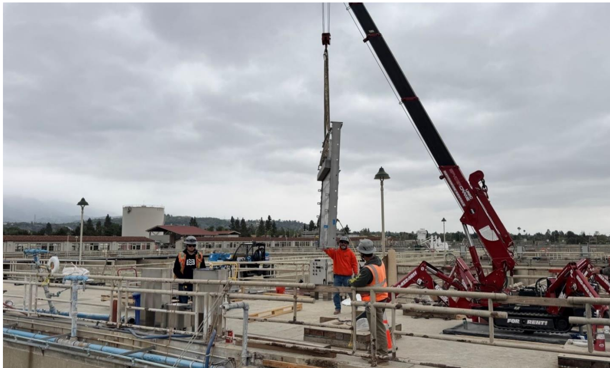
Hoisting a new inlet gate during installation at Basin No. 3
