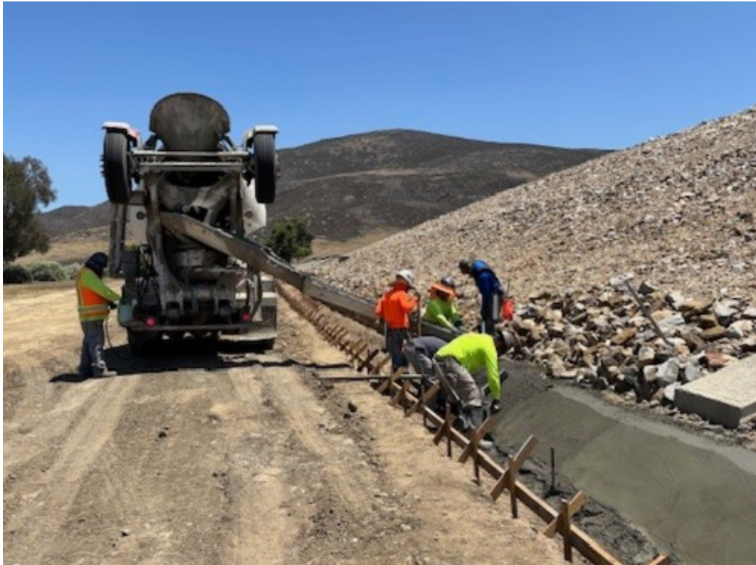
Lake Skinner Drainage Improvements – Placing Concrete V-Ditch
