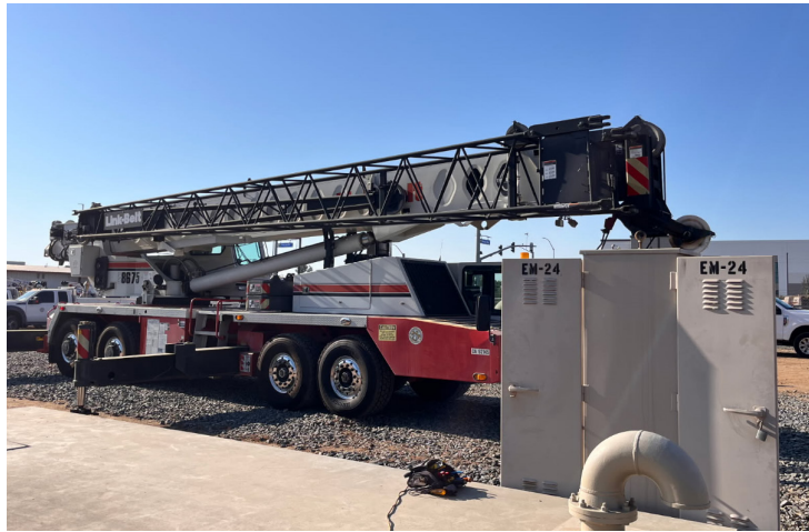
Crane on-site waiting to lift new flowmeter in place at EM-24
