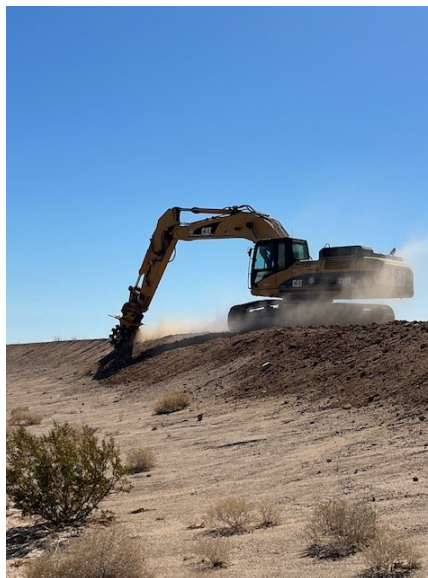
Staff repairing road banks and erosion areas near Eagle Mountain pump plant
