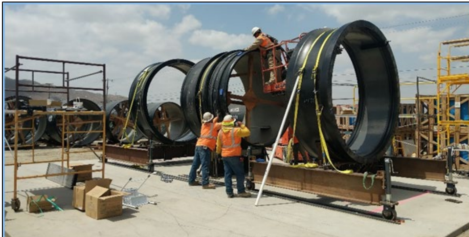
Figure 4-7: Earthquake Resistant Ductile Iron Pipe Joint Assembly for Casa Loma Siphon
