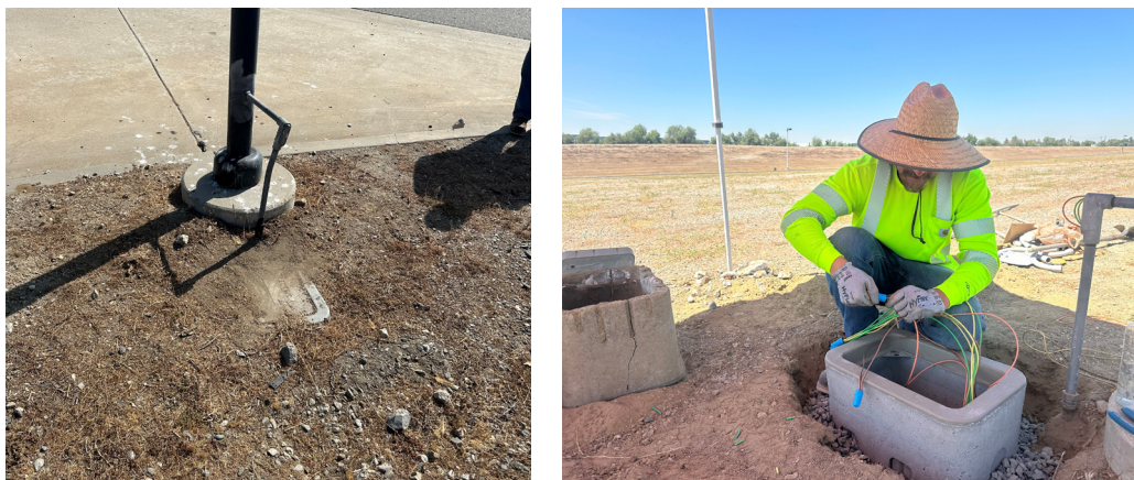
A buried pull box (left) and staff making repairs to a new raised unit (right) at Etiwanda HEP
