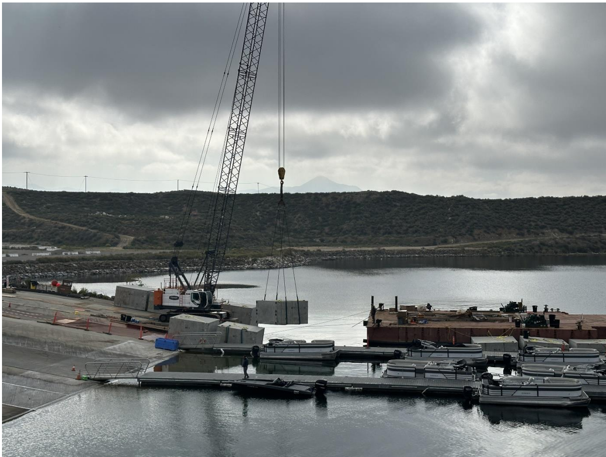
Lifting a floating wave attenuator module at Diamond Valley Lake
