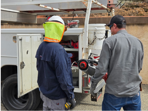
Threading conduit for installation (left) and conduit placement (right)
