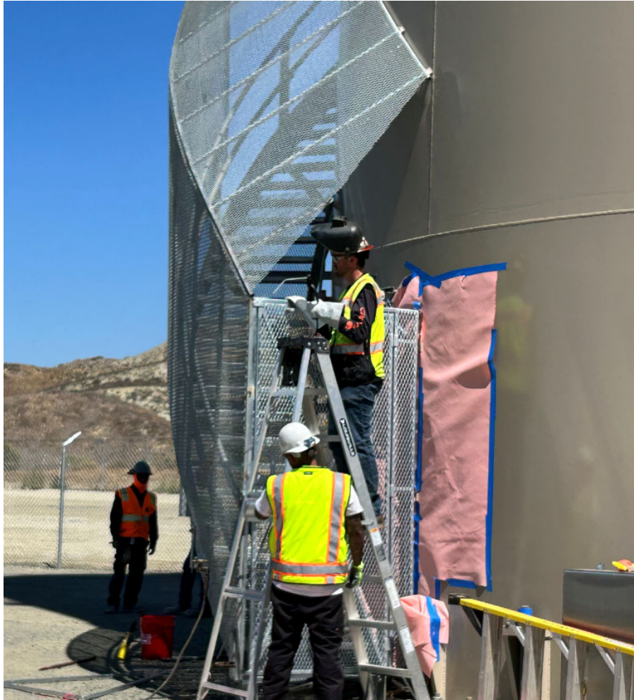
Inland Feeder-Badlands Tunnel Surge Protection – Spiral Staircase Door Installation
