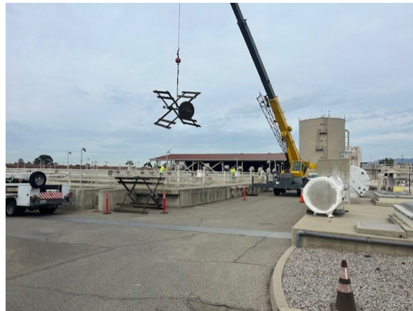
Damaged equipment, fabricating new stainless-steel stub shafts & replacement of equipment
