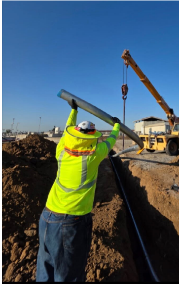
Staff installing conduit with crane support (left) and completed installation (right)
