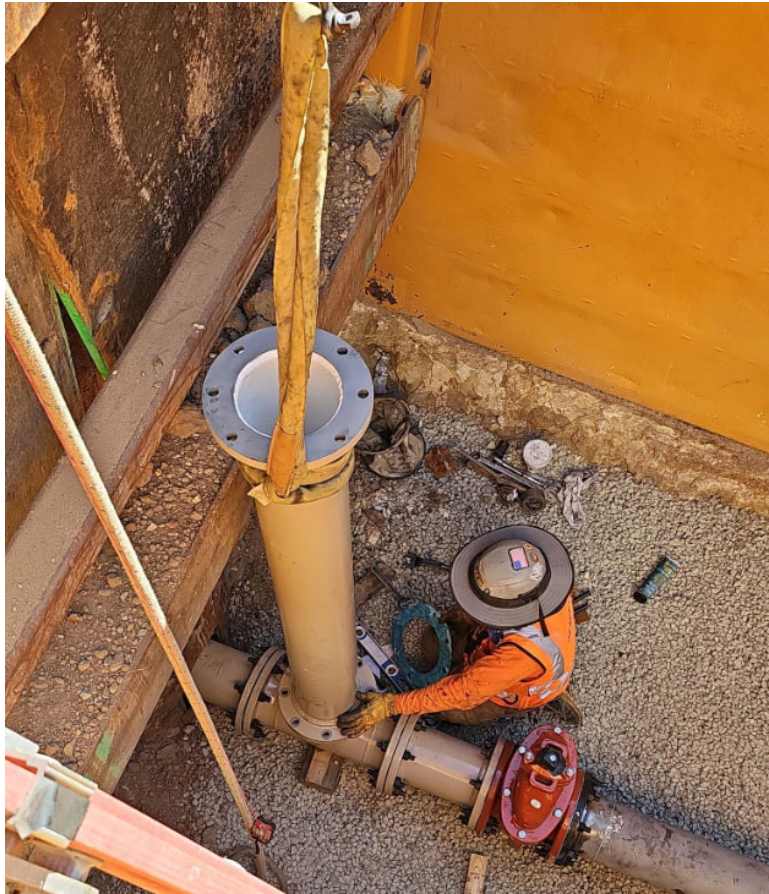
Second Lower Feeder PCCP Rehabilitation Reach 3B — Installing Mechanical Piping for Helopod Water Source
