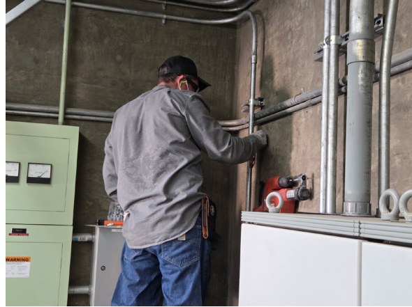
Threading conduit for installation (left) and conduit placement (right)
