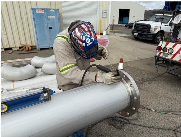
Staff welding stainless-steel piping
