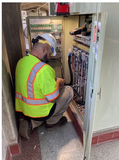
Staff working on wiring new valves at the valve control cabinet.
