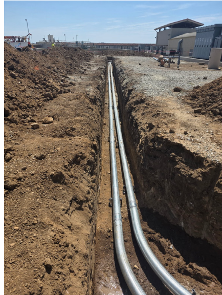
Staff installing conduit with crane support (left) and completed installation (right)
