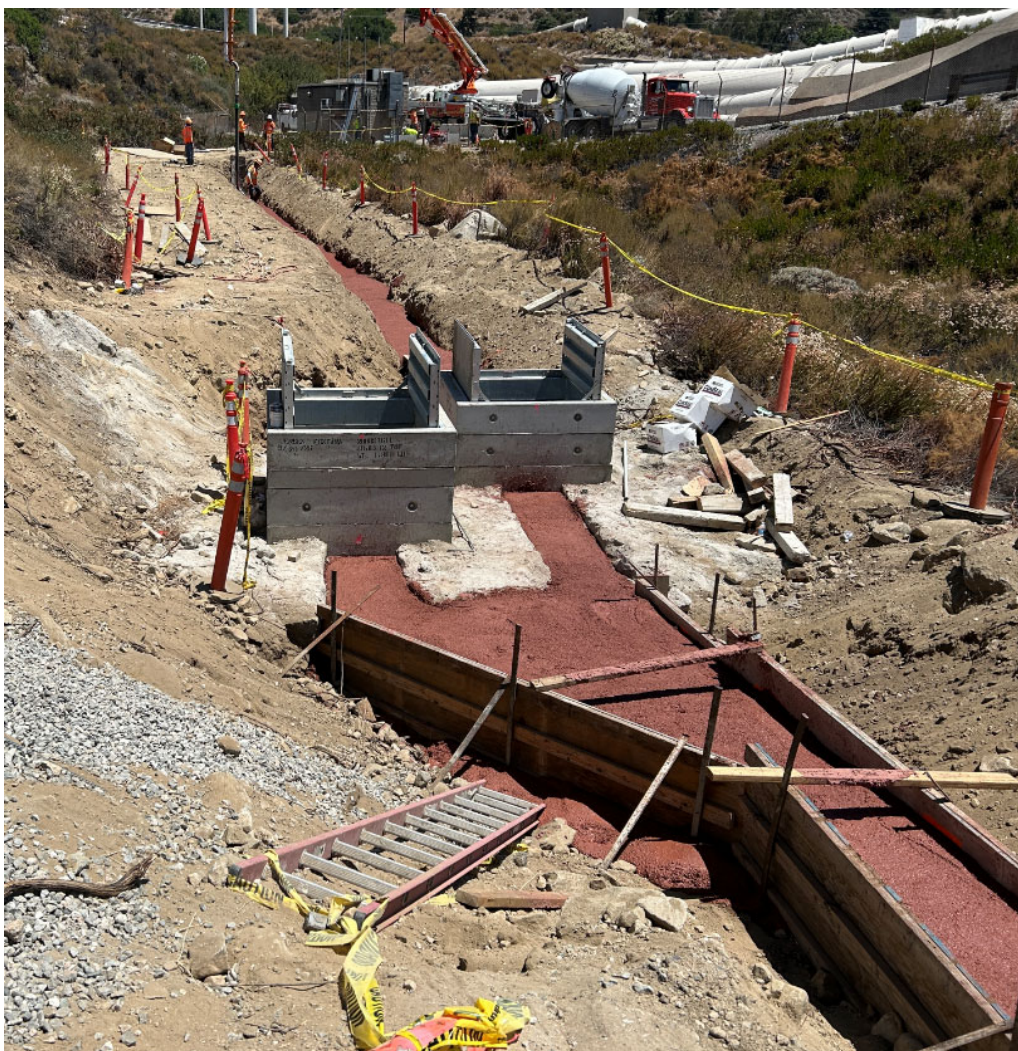
Inland Feeder Rialto Pipeline Intertie — Electrical Duct Bank Encasement Looking North
