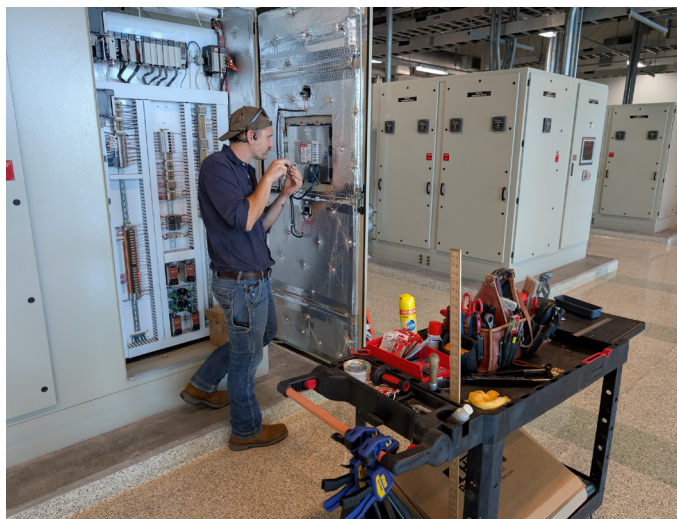
Staff is wiring a new HMI screen for a power supply unit.
