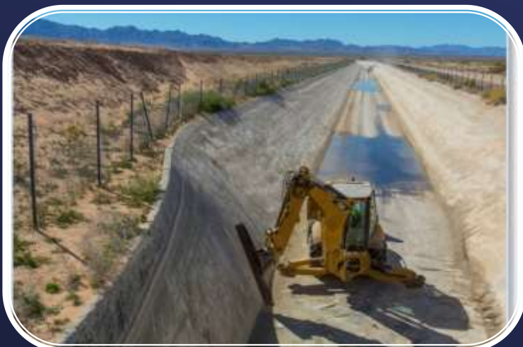
Desiccation, Cleaning and Inspections during CRA Shutdowns
