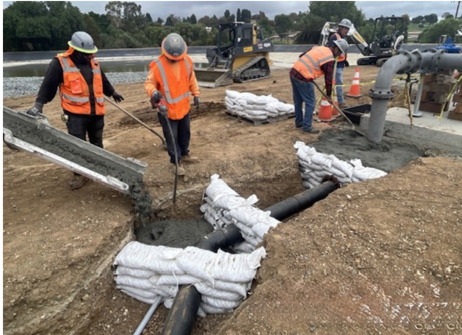
Second Lower Feeder PCCP Rehabilitation Reach 3B — Palos Verdes Reservoir Placing Concrete Thrust Blocks for Helopod
