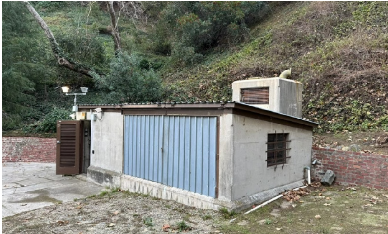
Hollywood Tunnel North Portal Control Structure
