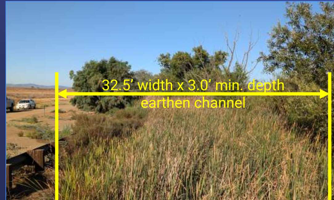
Holland Road Earthen Channel
