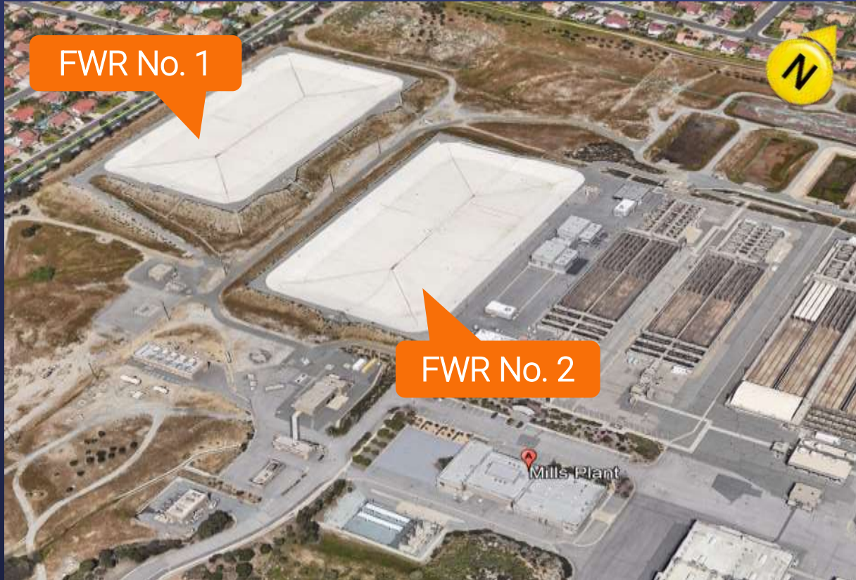
Henry J. Mills Water Treatment Plant
