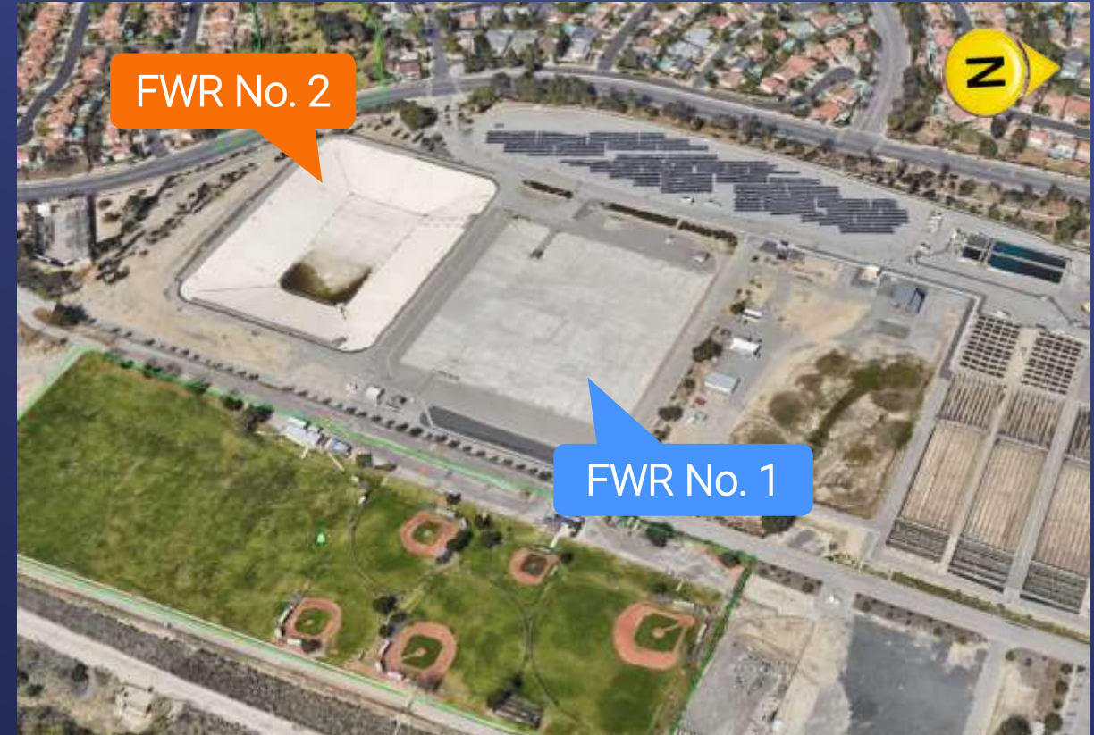
Joseph Jensen Water Treatment Plant
