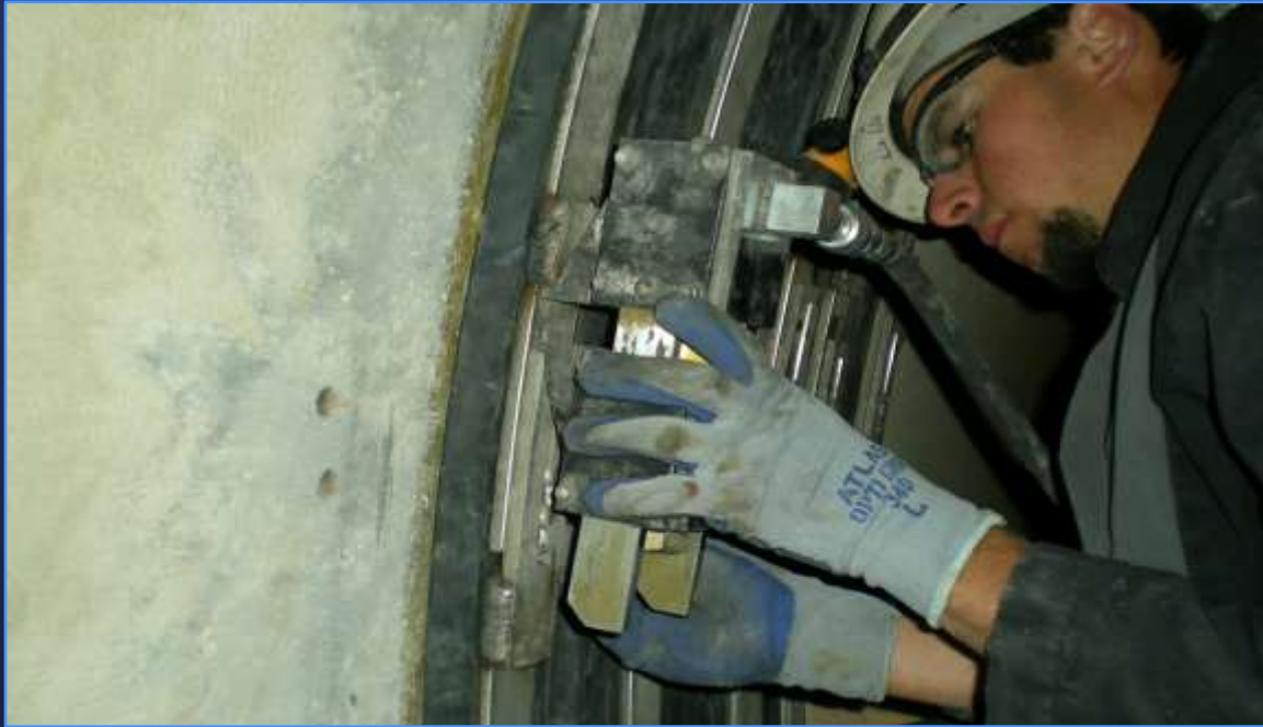
Seal Installation
