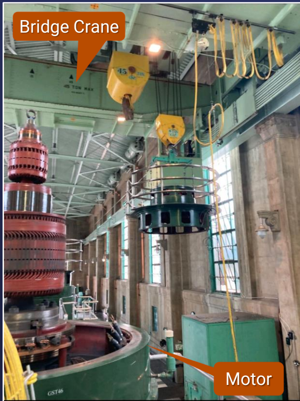
Overhead Crane in Use
