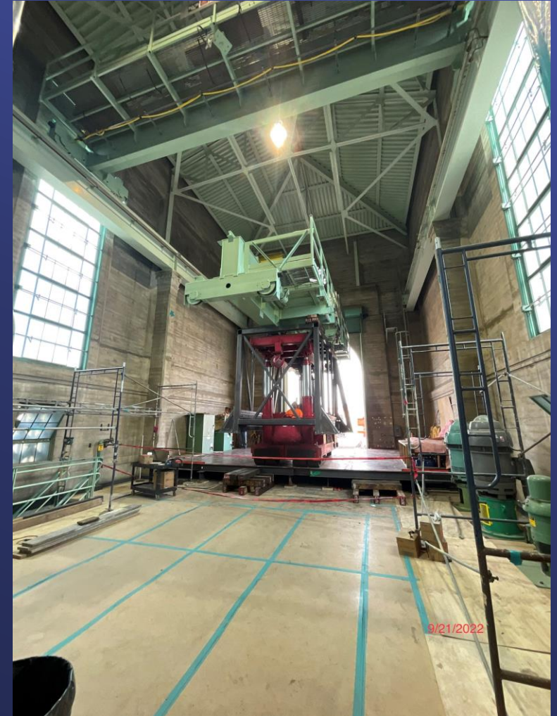
New Crane Girder Installation @ Gene
