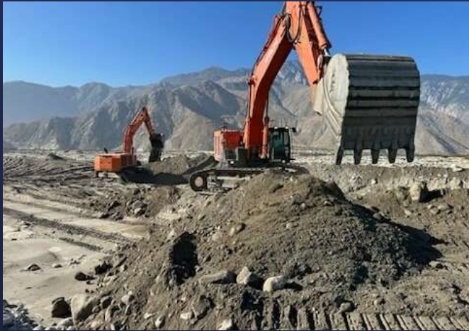
Metropolitan staff repairing Main Channel
