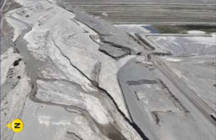
Damage to Earthen Channel
