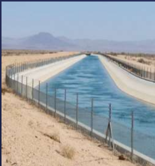
Colorado River Aqueduct
