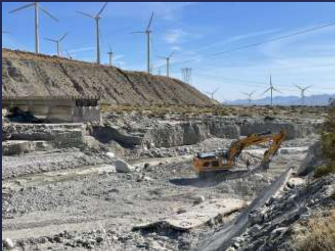
Whitewater Bridge Demolished
