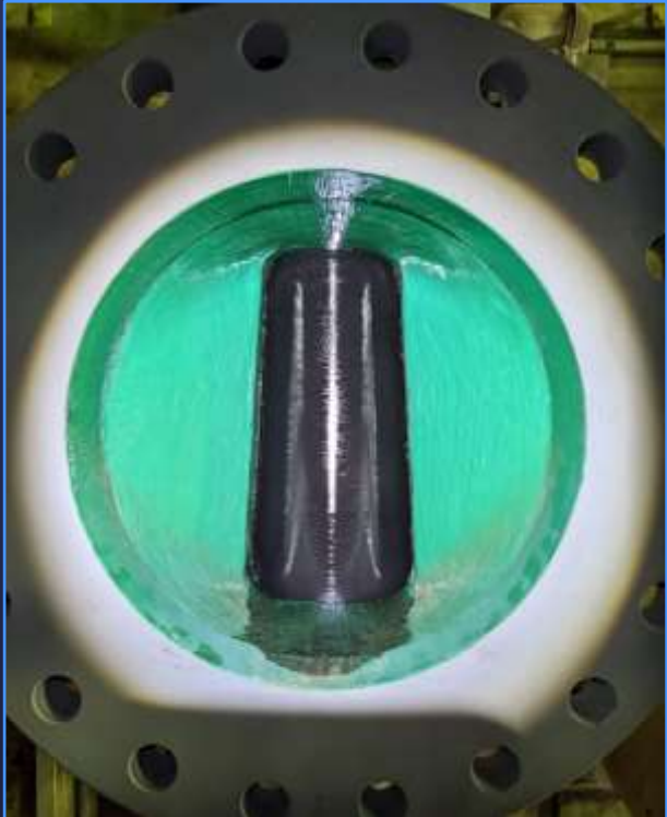
New Plug Valve Interior
