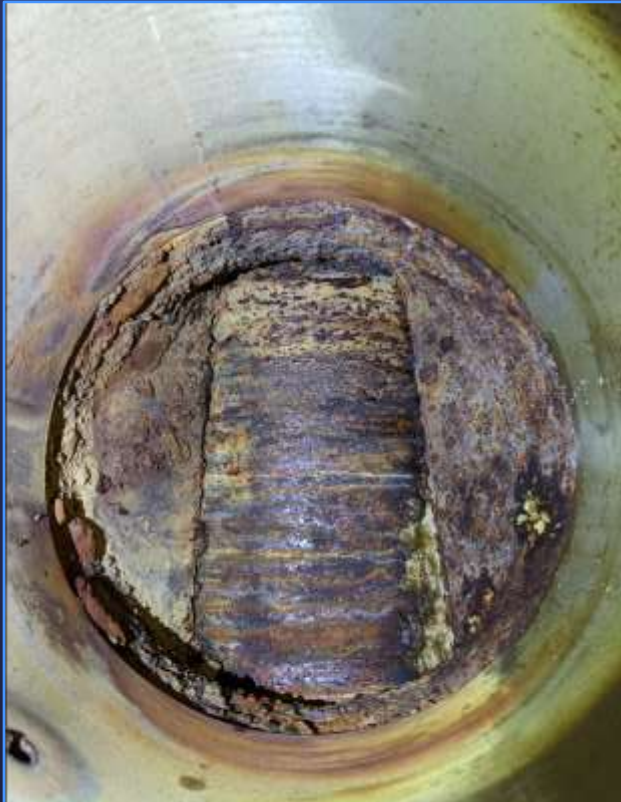
Existing Plug Valve Interior
