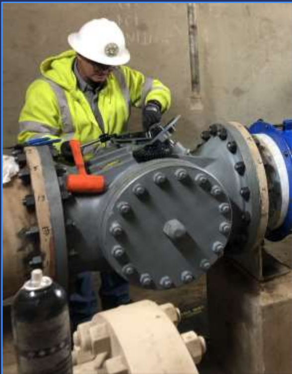
Plug Valve Installation
