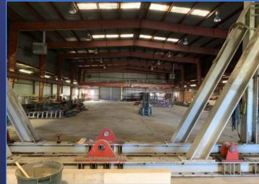
Pre-Phase 1 CSI Building
