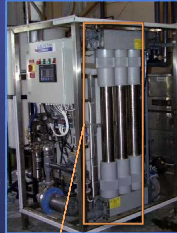
Existing Microfiltration Units
