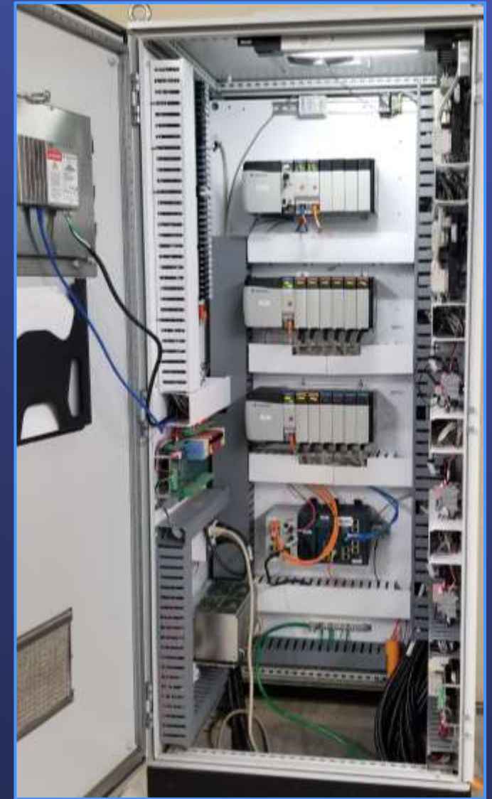
PLC Panels (Typical)
