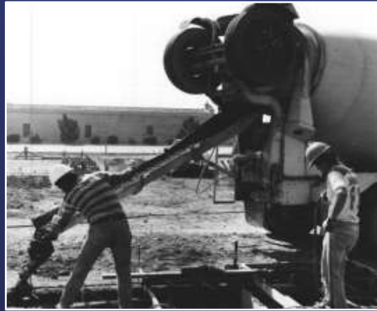
Pouring concrete for Water Quality Lab, 1983
