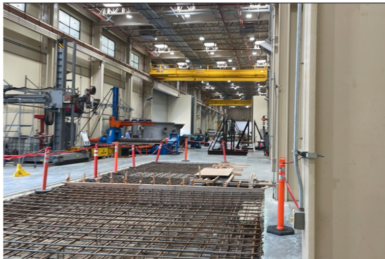
Installation site for the new MSU Shop Plasma/Oxy-Fuel Cutting System
