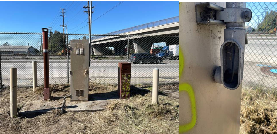
Reinforced AMR meter cabinets eliminate monitoring outages due to metal, power, and UPS battery thefts
