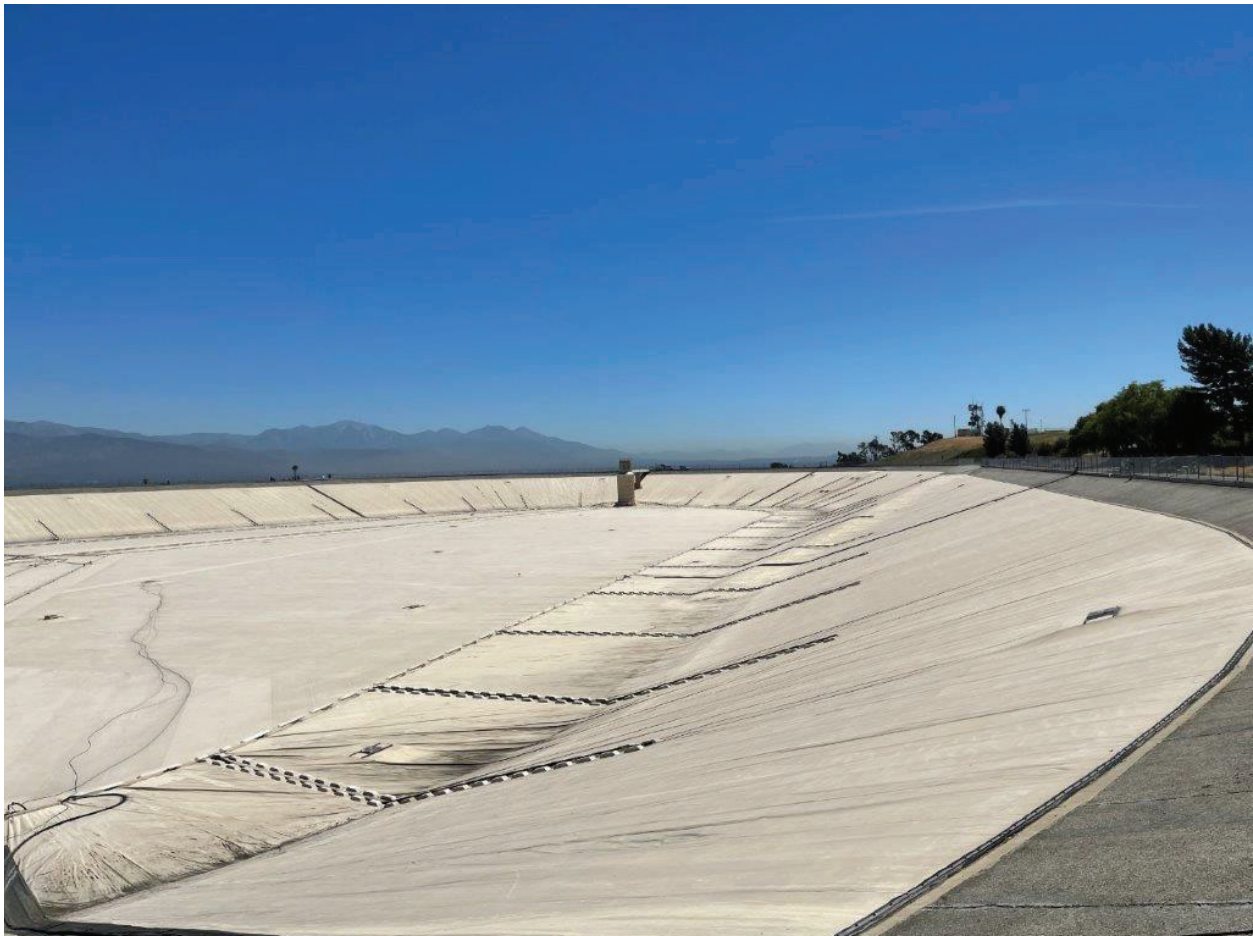
View of the existing Garvey Reservoir floating cover
