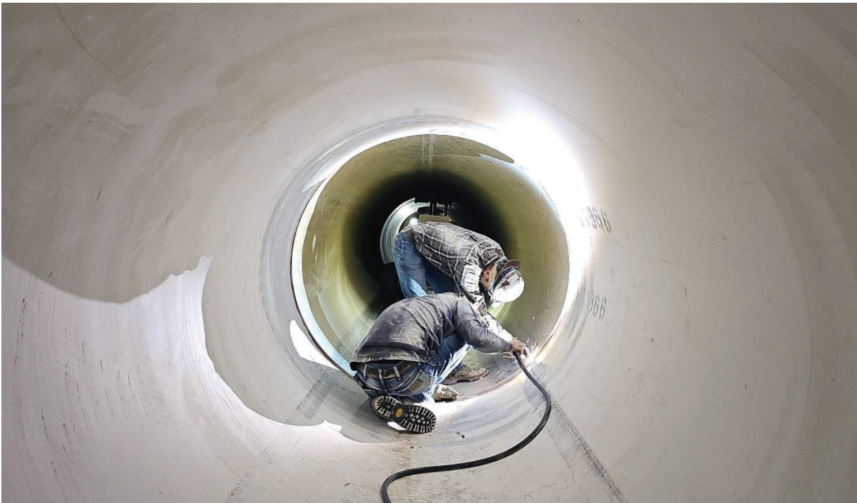
Welding pipe connection for AMP, Stage 1
