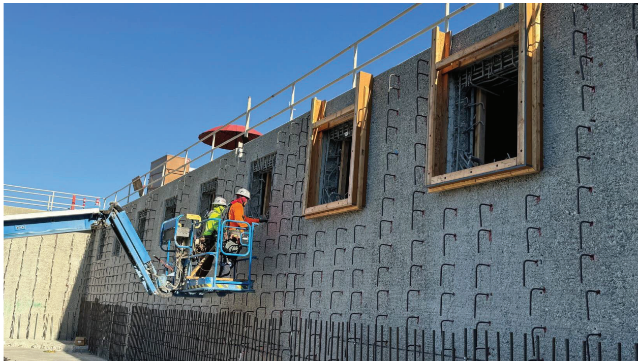
Setting launder blockouts at Weymouth Water Treatment Basin No. 6
