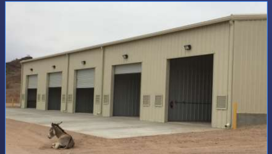
Gene Storage Building (New)
