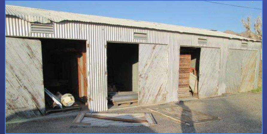
Iron Mtn. Storage Building (Existing)
