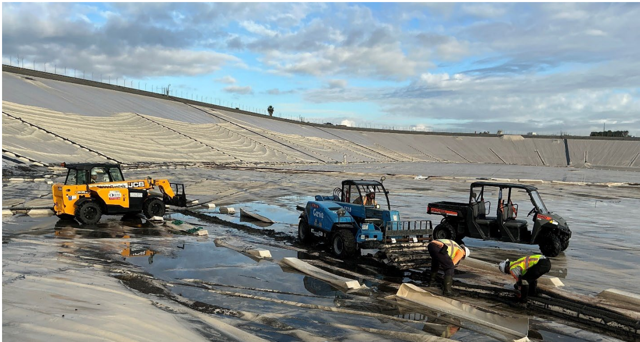
Demolition of reservoir cover rainwater collection system at Garvey Reservoir
