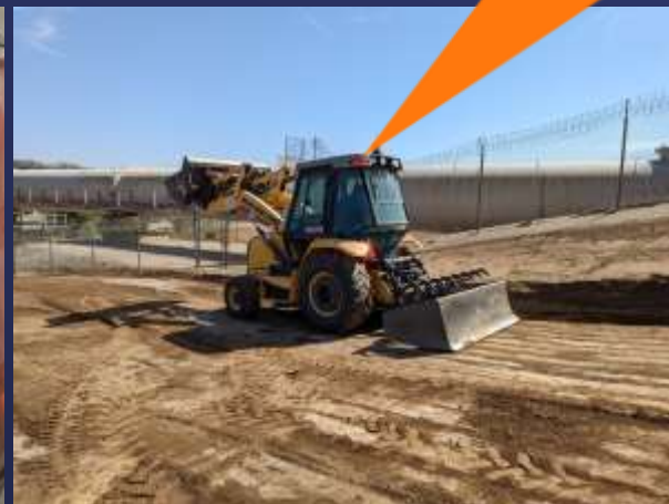
Clearing and Grading for Crane Pad
