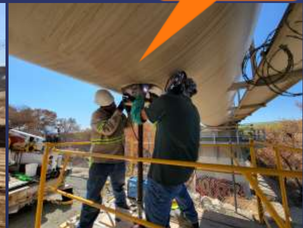
6-inch Valve Installation
