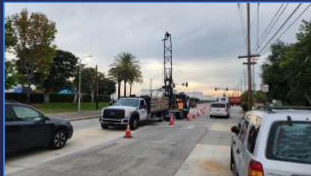
Pure Water Conveyance Reach 1 Utility Investigation
