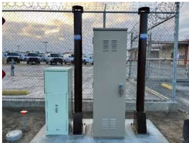
The repaired CenB-49 metering station
