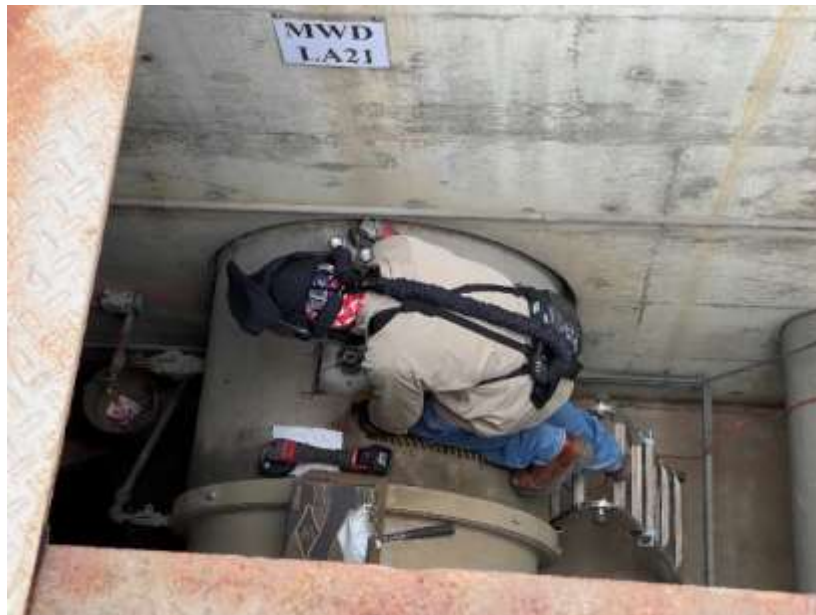
Staff performing hot tap at the LA-21 service connection
