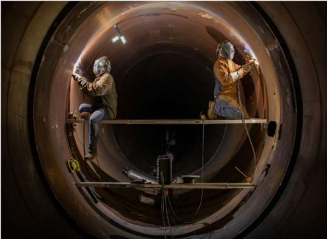
Etiwanda Pipeline Relining—Welding Steel Pipe Reducers
