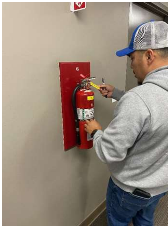
Staff performing inspection of a fire extinguisher at the Diemer plant
