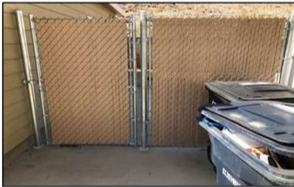
Fencing Privacy Slat Installation at Iron
