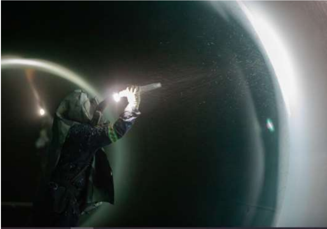
Etiwanda Pipeline Relining—Applying Polyurethane Coating Lining
