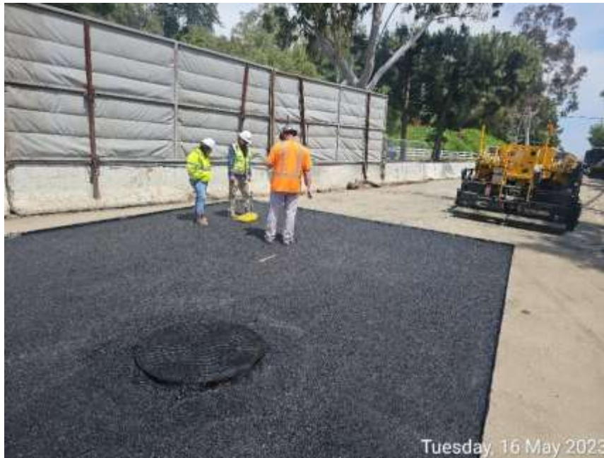
Second Lower Feeder PCCP Rehabilitation Reach 3A—Street Restoration
