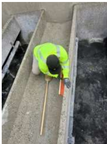
Staff finishing filter cleaning at the Jensen plant
