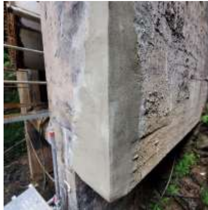
Concrete repair of Copper Basin discharge valve structure
