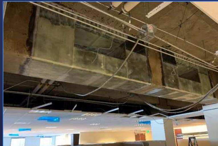
Interior Beam with Fiber Reinforced Polymer (FRP)
